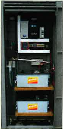
Solar mechanics accessed through rear panel
