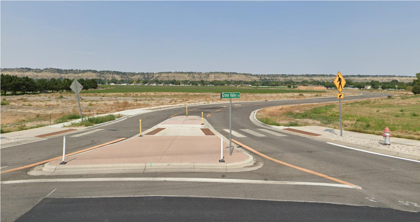
Intersection of Green Valley Drive at Grand Avenue
