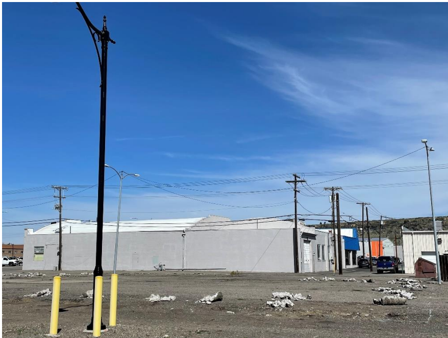
Ice Plant Site at 1523 Montana Avenue looking North from Montana Avenue.
