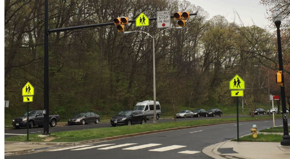
Pedestrian hybrid beacon on a divided roadway
