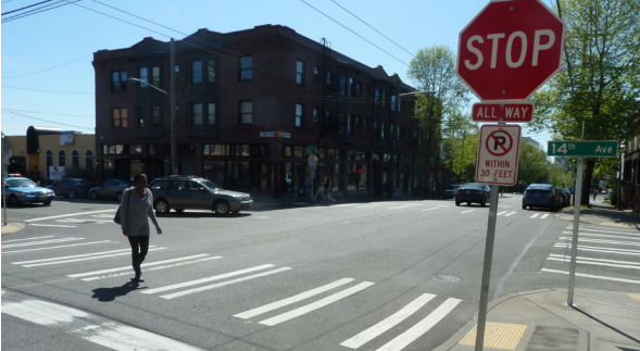
Stop sign with stop line at an all-way stop
