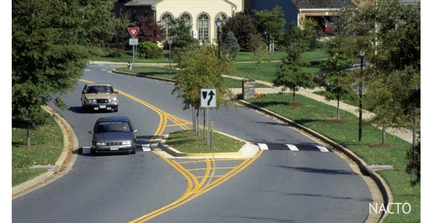
Speed humps installed on hills help slow traffic coming downhill
