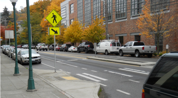
Mid-block curb extension
