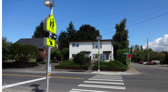
RRFB with push button at a school crosswalk
