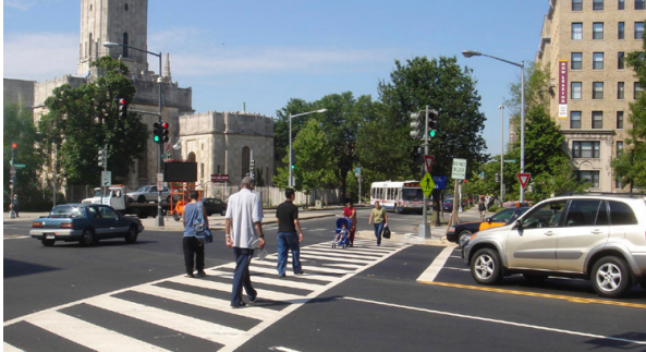
Marked ladder style crosswalk at an intersection
