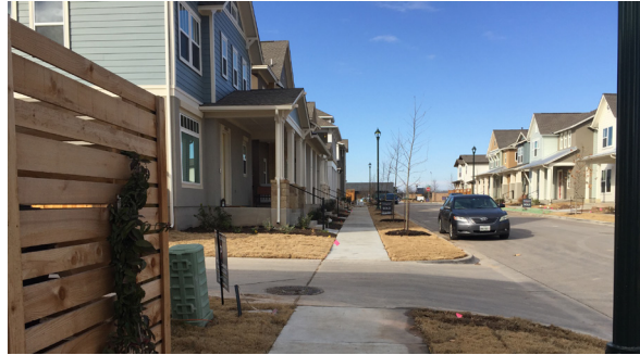
New sidewalk remains level across driveway
