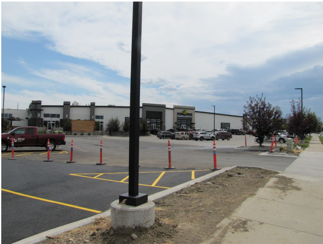
View west along Gabel Road
