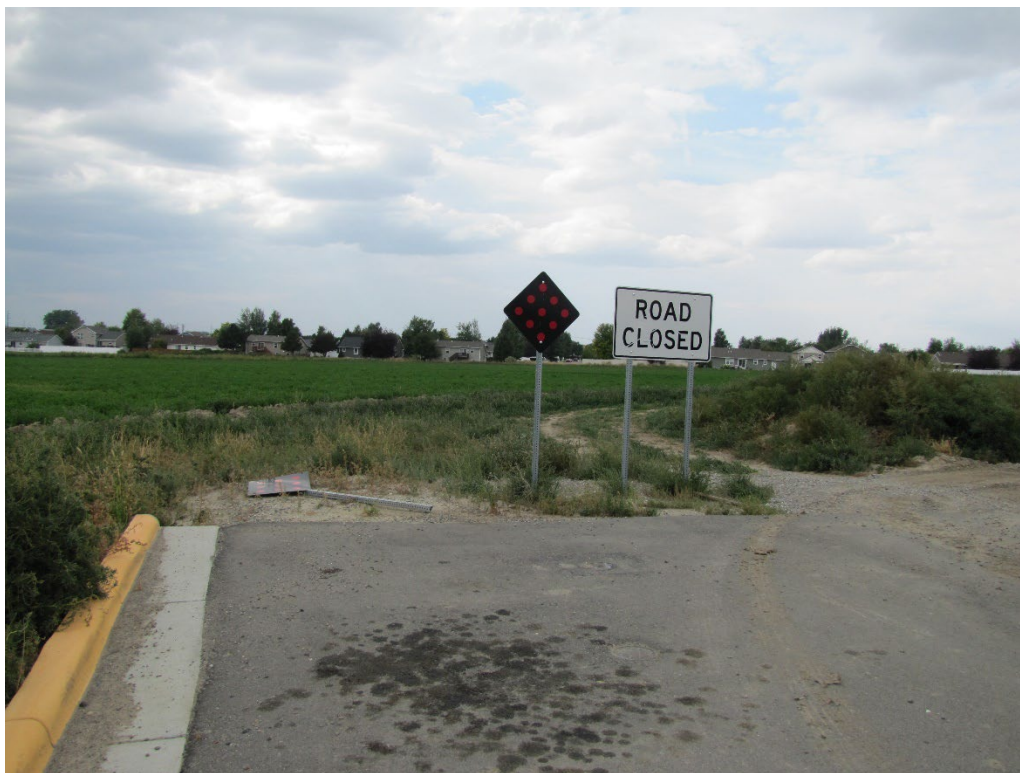
Dead end of Avenue D – north east property corner
