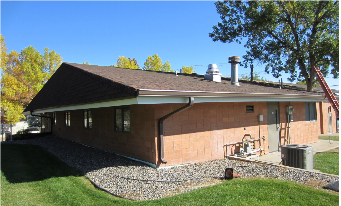
OVERVIEW OF SOUTH WEST EXPOSURE
