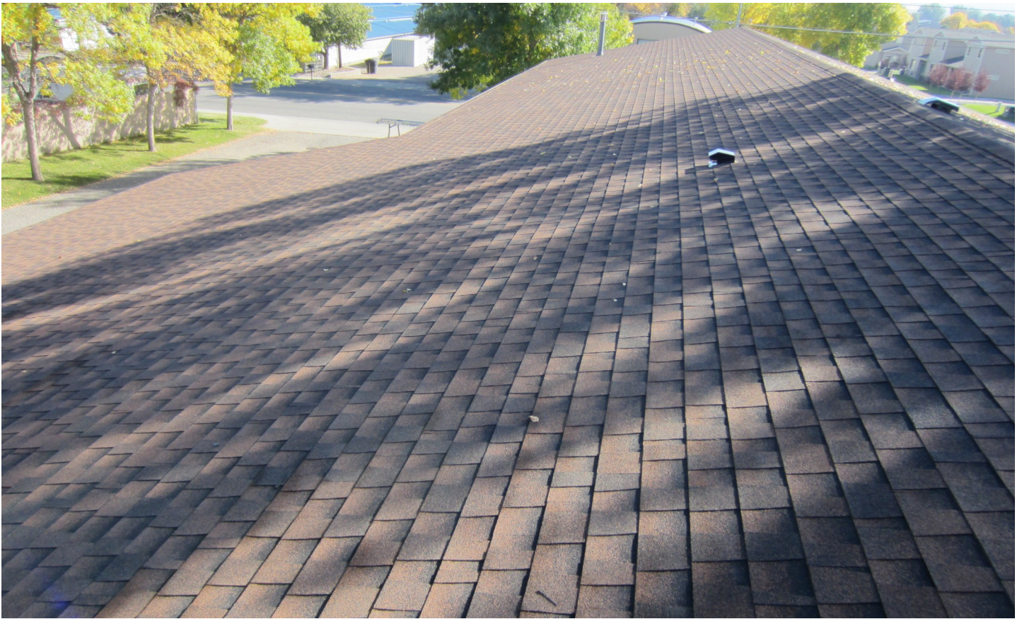
OVERVIEW OF NORTH SIDE OF ROOF LOOKING EAST.
