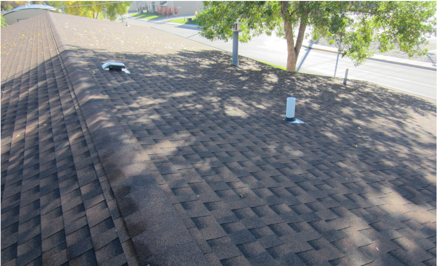
OVERVIEW OF SOUTH SIDE OF ROOF LOOKING EAST.
