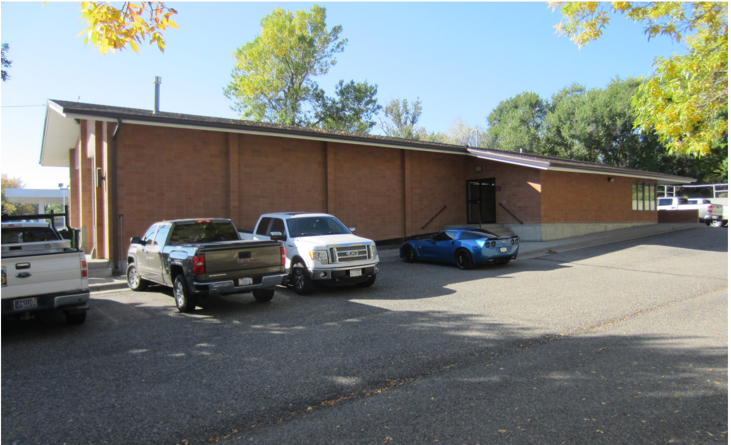
OVERVIEW OF NORTH SIDE
