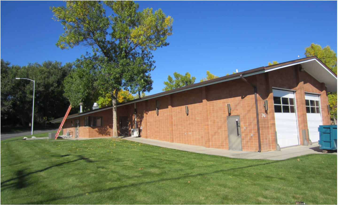
OVERVIEW OF SOUTH SIDE
