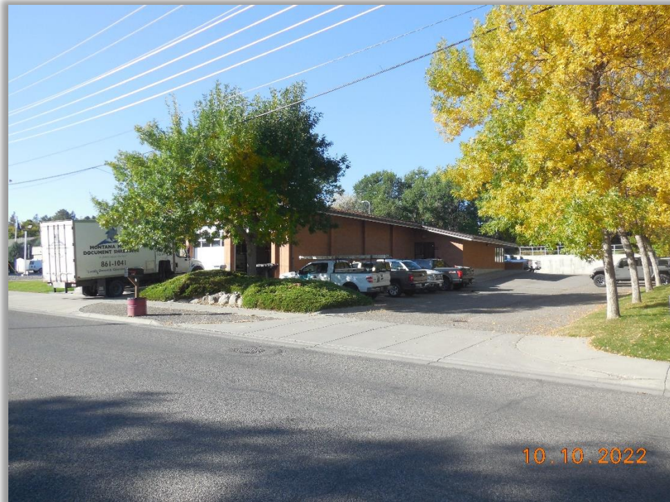
The east and north elevations of the subject property looking to the southwest Taken by Matt Bender
