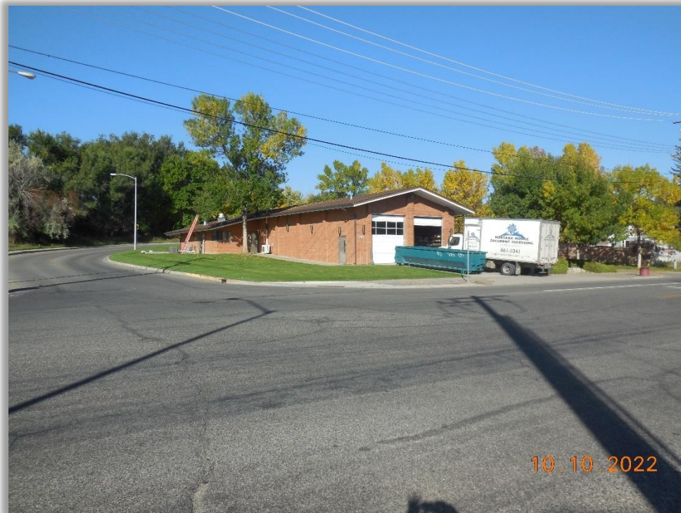
The south and east elevations of the subject property looking to the northwest Taken by Matt Bender
