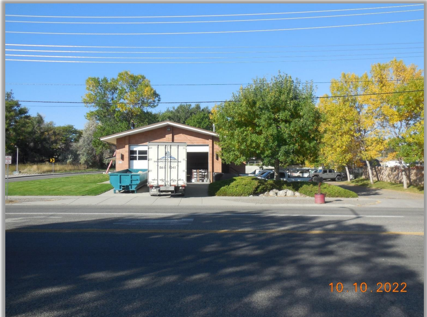
Office Building 760 Lake Elmo Dr. Billings, Montana
