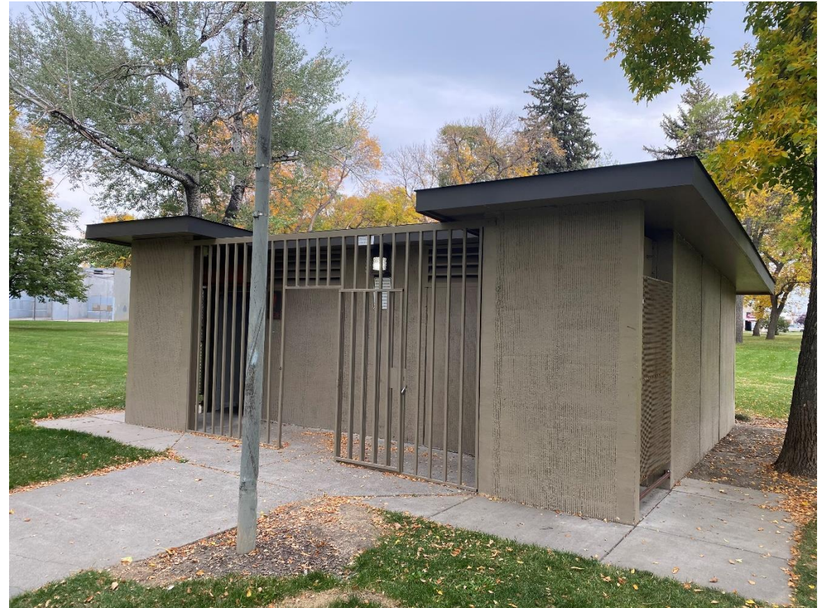
Current Restroom at North Park
