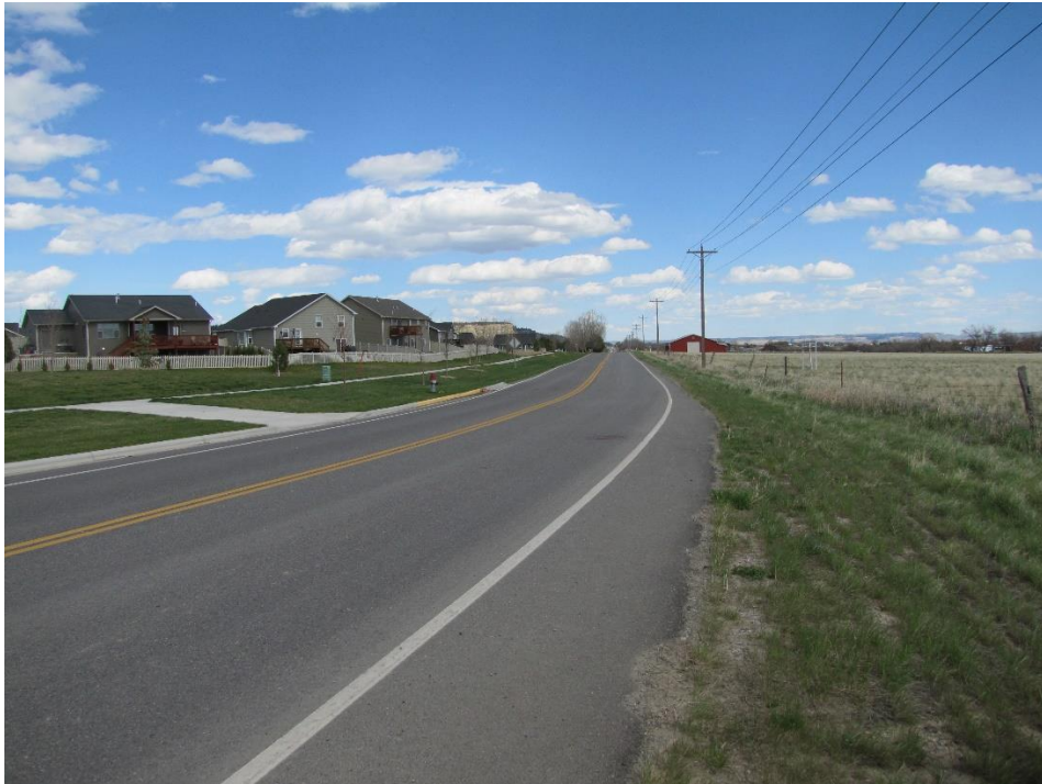
View east on Rimrock Road
