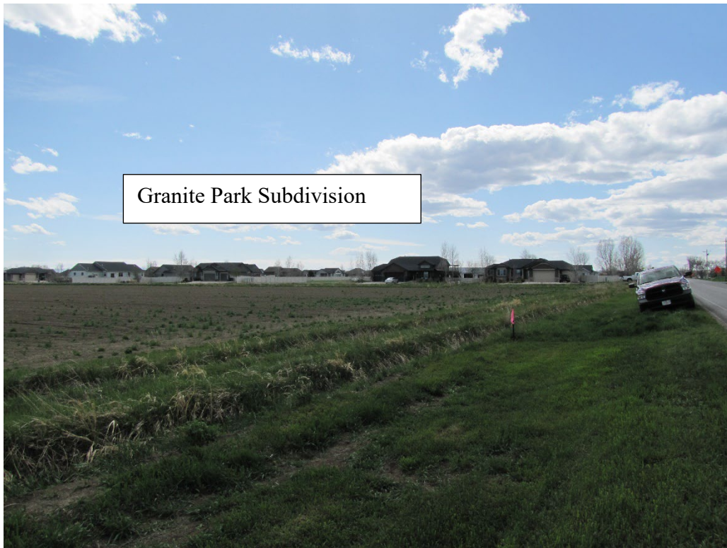
View west along Central Avenue
