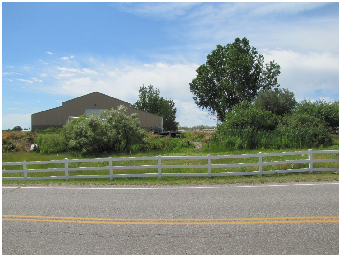
View west across Bitterroot Drive
