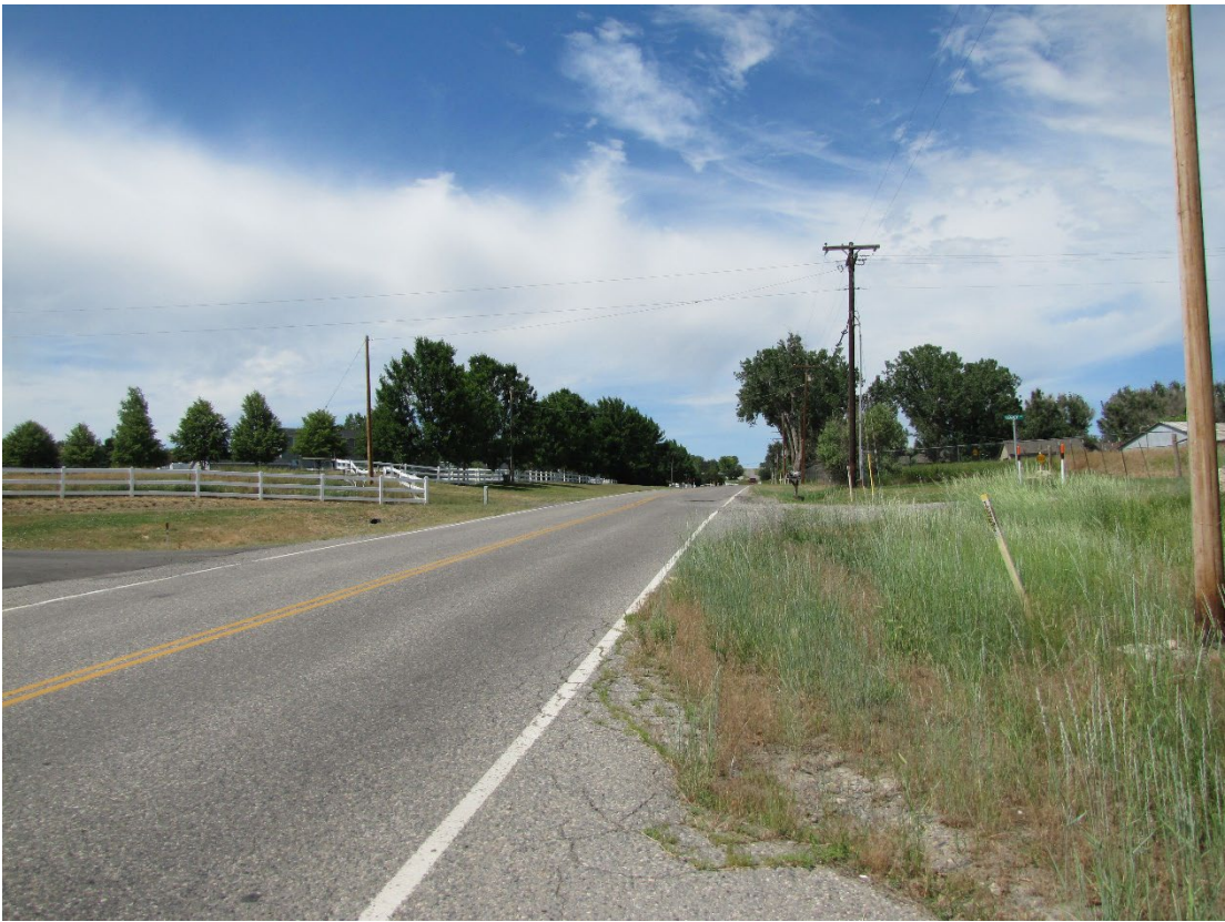
View north and west across Bitterroot Drive
