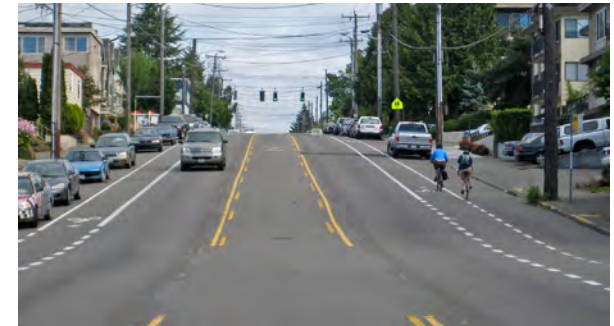
Center turn lane narrowed to provide space for bike lanes
