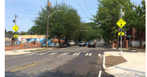
RRFB at a neighborhood bikeway crossing
