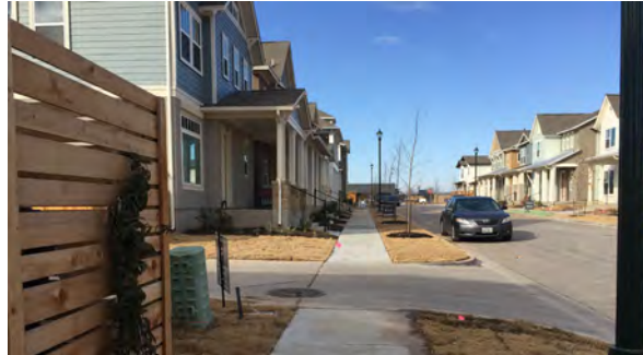
New sidewalk remains level across driveway
