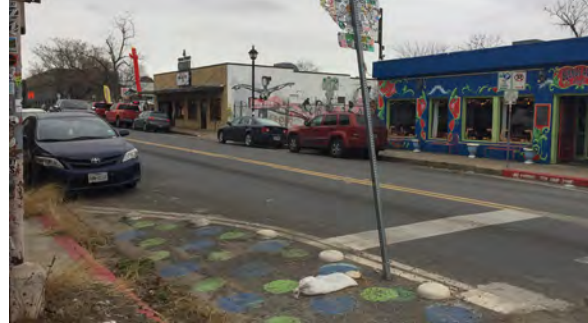
Easy-to-install materials such as paint, turtle bumps, and flex posts may be used to create curb extensions
