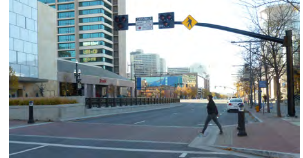
Pedestrian hybrid beacon on a downtown street
