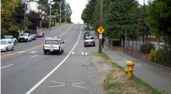
Street before lane reconfiguration
