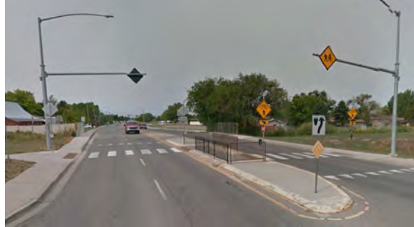
A pedestrian refuge island assists people crossing Broadwater Ave.
