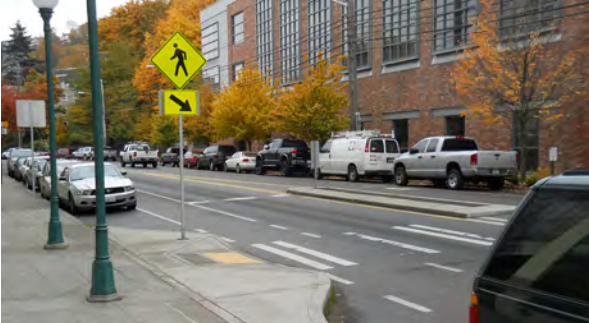
Mid-block curb extension
