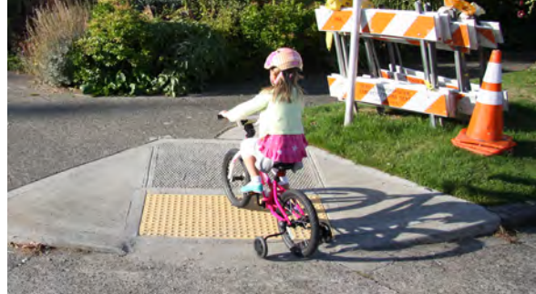
A sidewalk retrofitted with a curb ramp and a tactile warning strip
