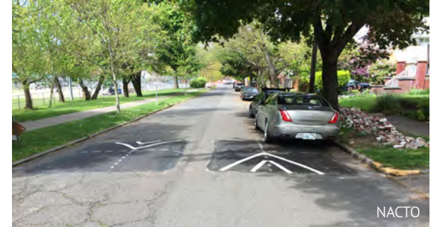
Speed cushions installed on hills may include a cut for downhill bicyclists
