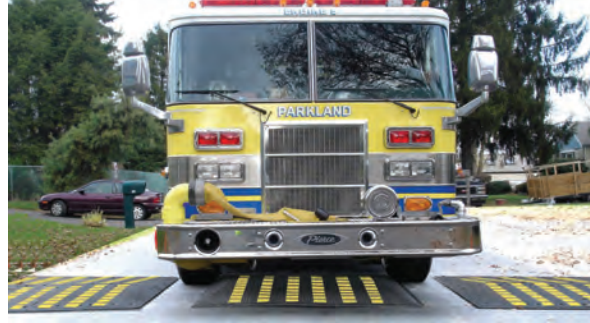
Speed cushions allow for larger vehicles such as fire trucks to pass through unimpeded
