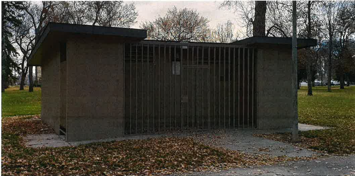
Subject of photo: North Park Restroom, Billings, MT 59101
