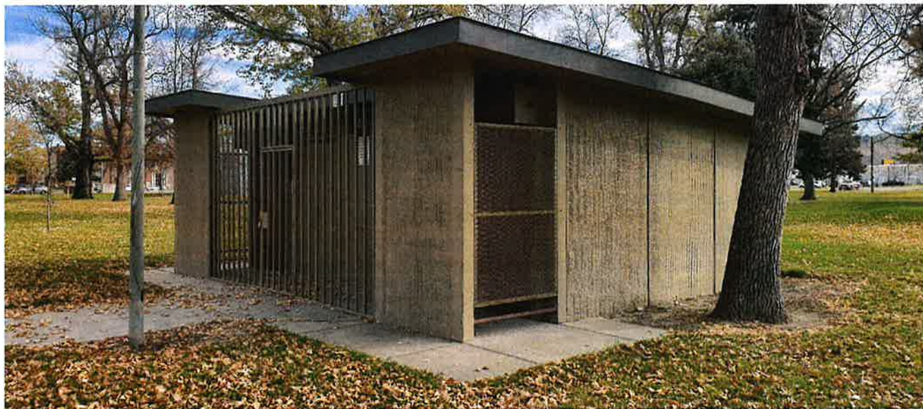
Subject of photo: North Park Restroom, Billings, MT 59101
