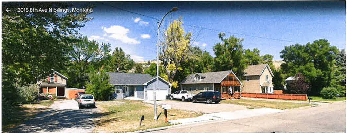
Subject of photo: Residential properties along 8 th Avenue N, Billings, MT 59101 Property across the street to the north of the subject property
