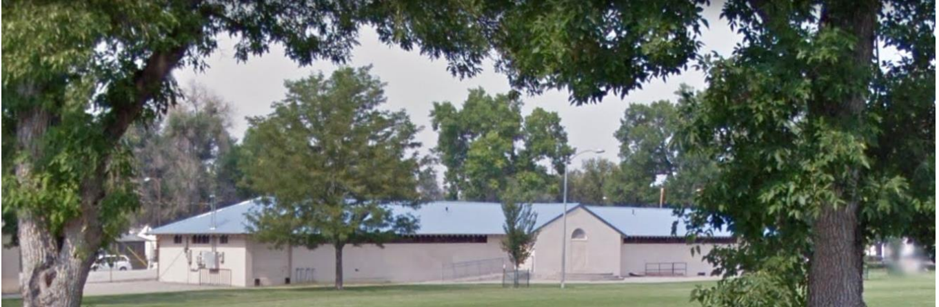
Subject of photo: South Park pool house, Billings, MT 59101 Photo Taken Looking: North
