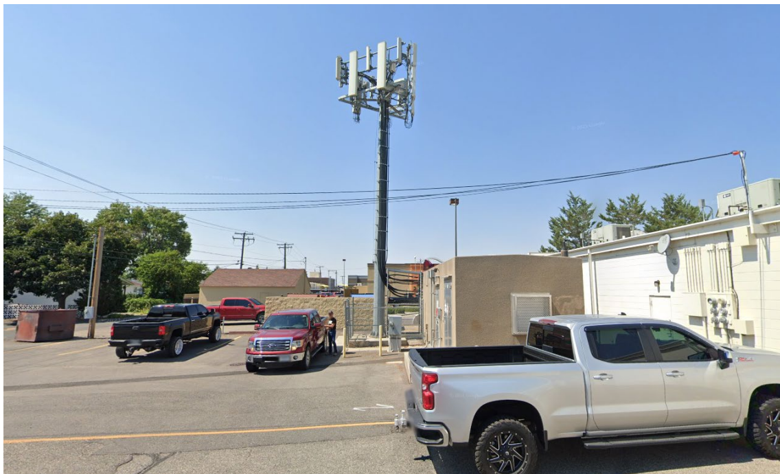
View west from 10 th St West
