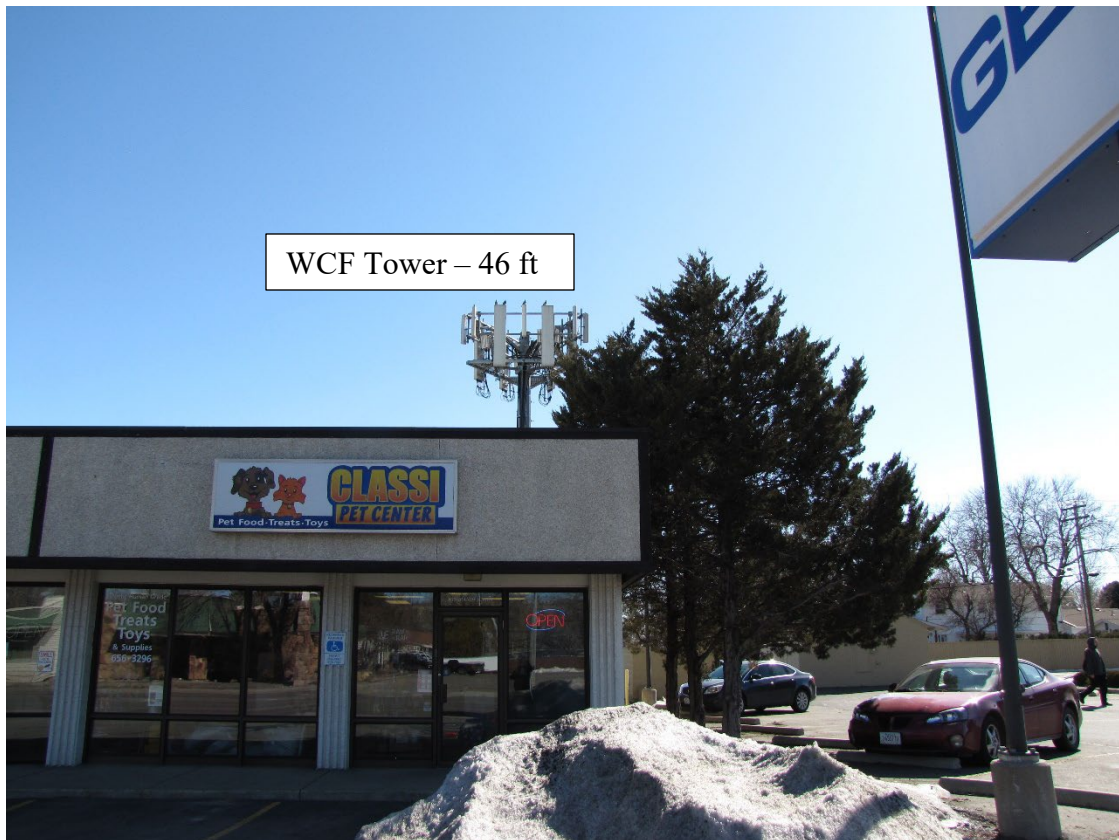
Subject Property – WCF tower
