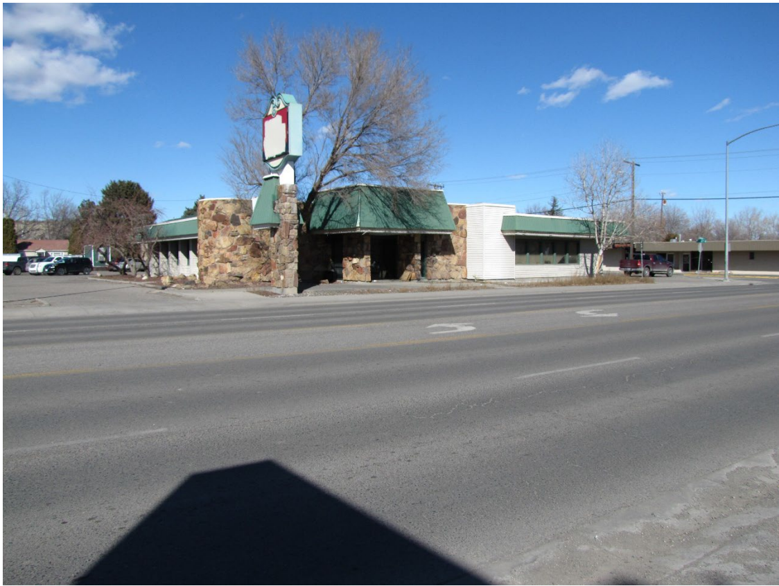
View north across Grand Avenue
