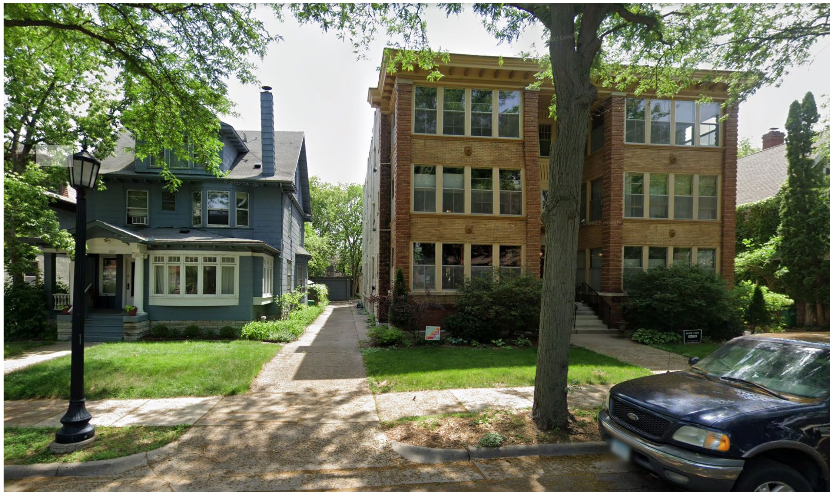
Humboldt Ave Minneapolis MN
