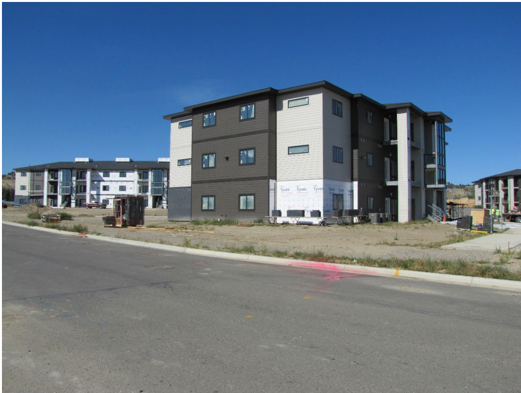
View northeast across Avenue E
