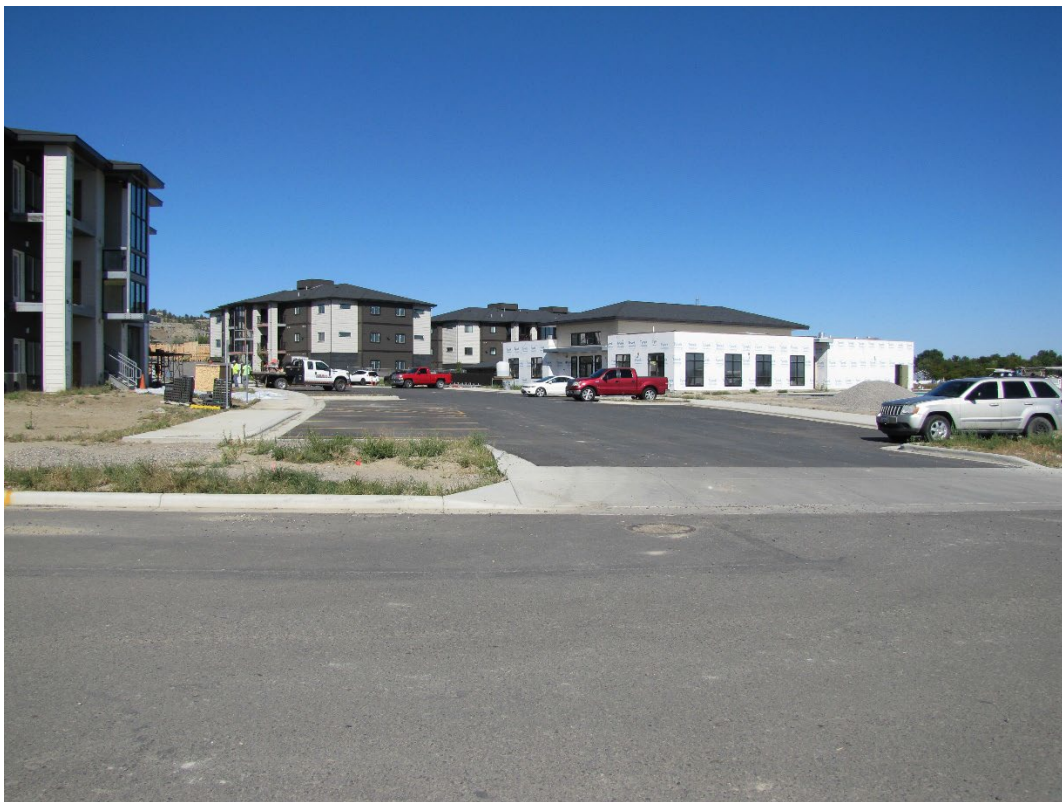
View east across Avenue E
