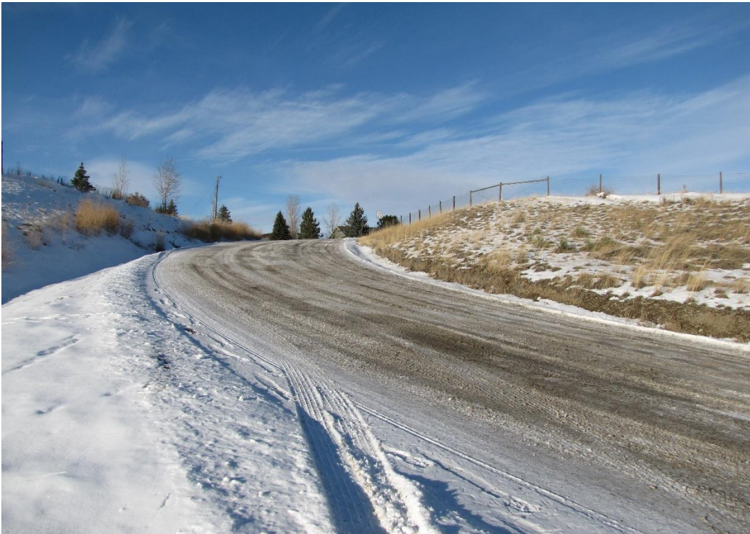
Looking North West on Basin Creek Rd.
