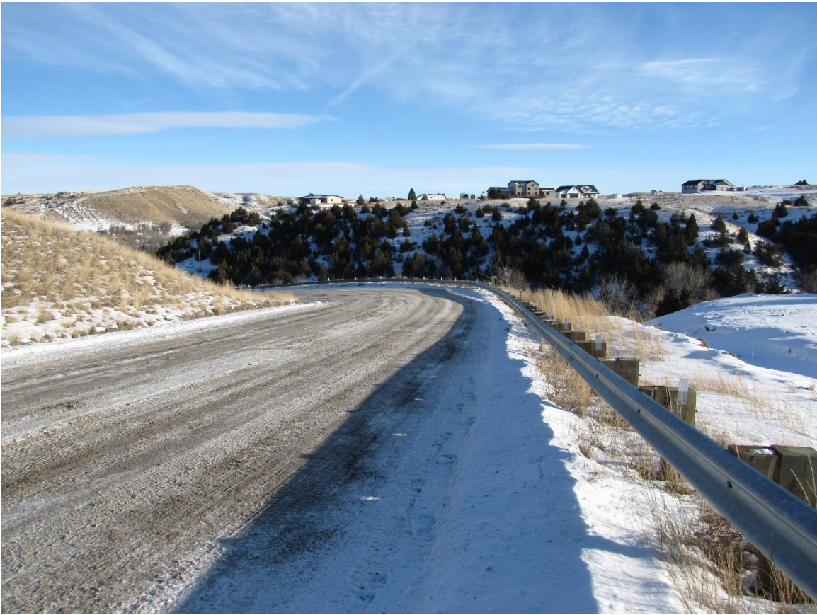
Looking South East along Basin Creek Rd.
