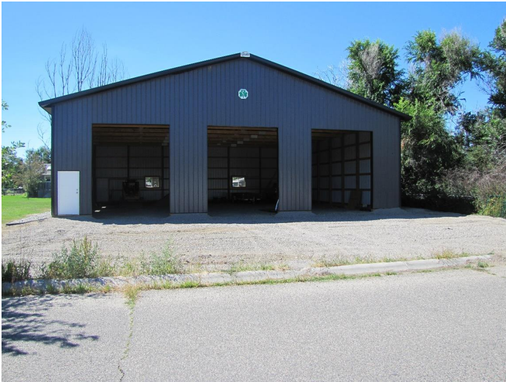
The 60x60 structure on Hawthorn
