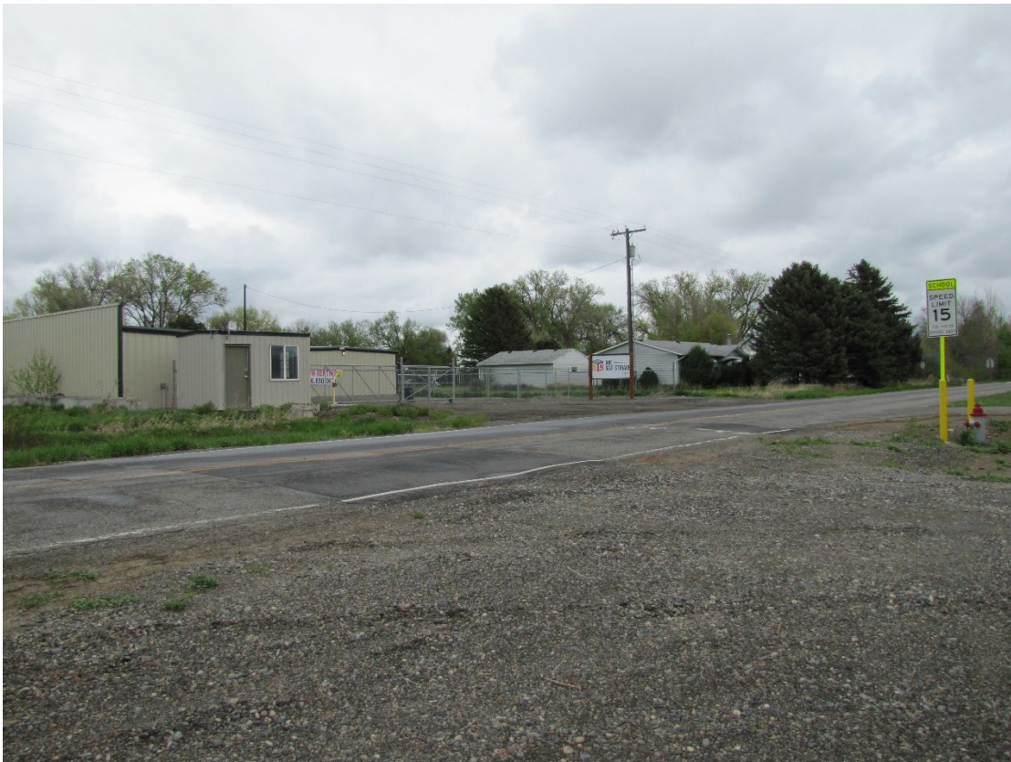
View north and east across Elysian Rd
