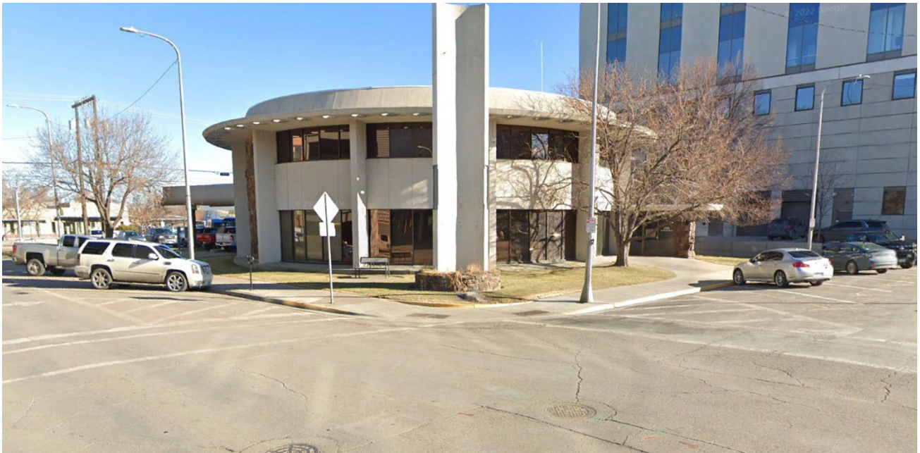
Subject Property view south east across 3 rd Ave N – prior to demolition
