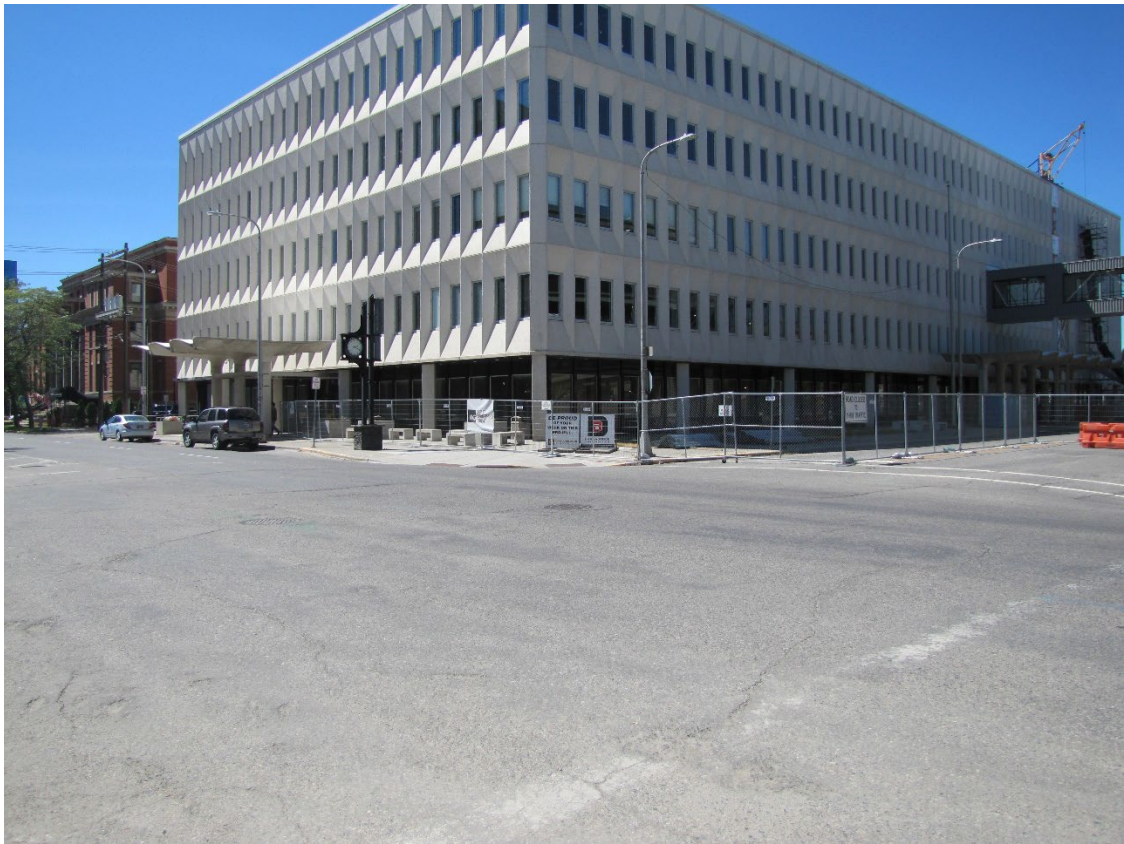
Stillwater Building aka new City Hall north west across 3 rd Ave N
