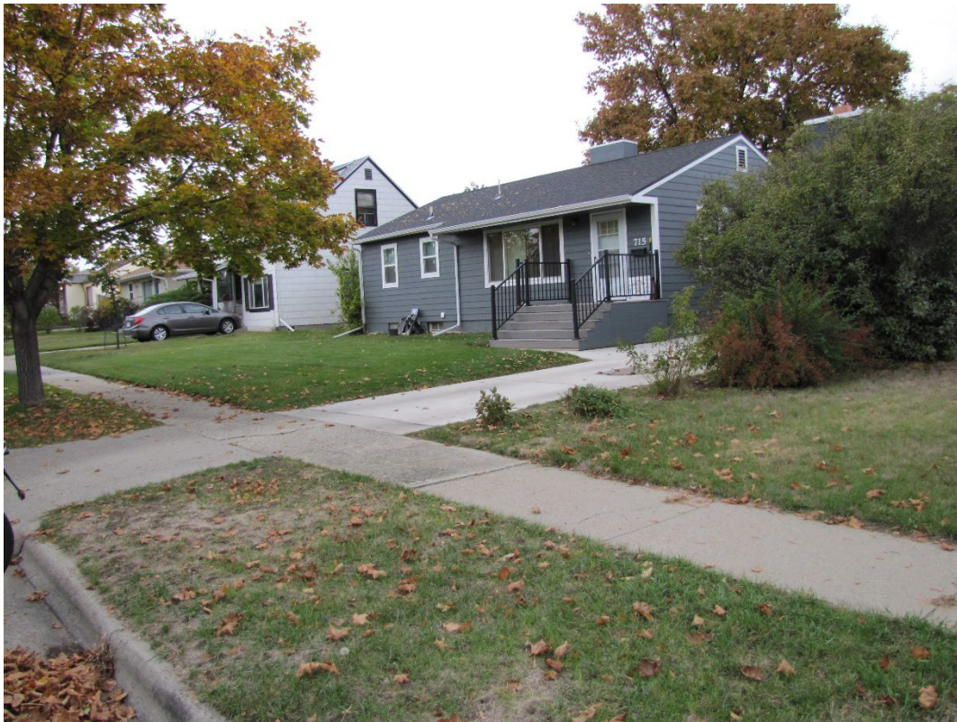
View north west to adjacent duplex at 715 Avenue D
