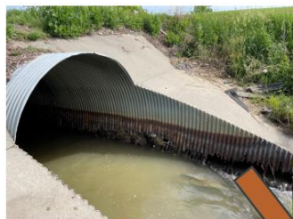
Corroded Culverts
