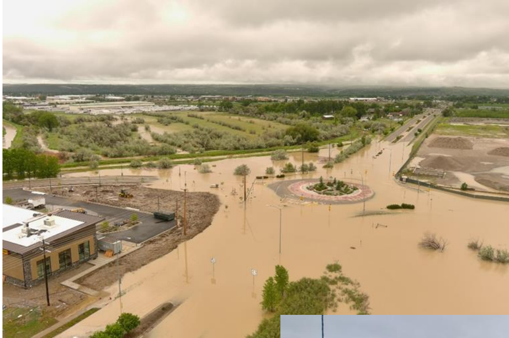
Shiloh Road Flooding
