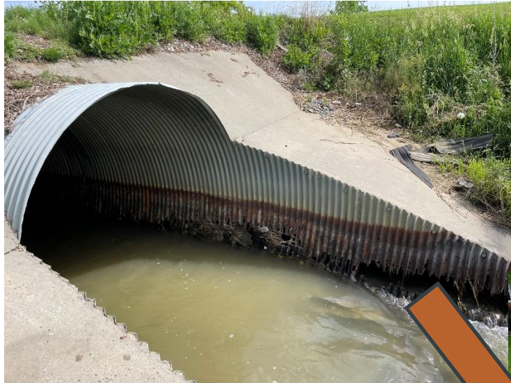
Corroded Culverts
