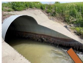
Corroded Culverts
