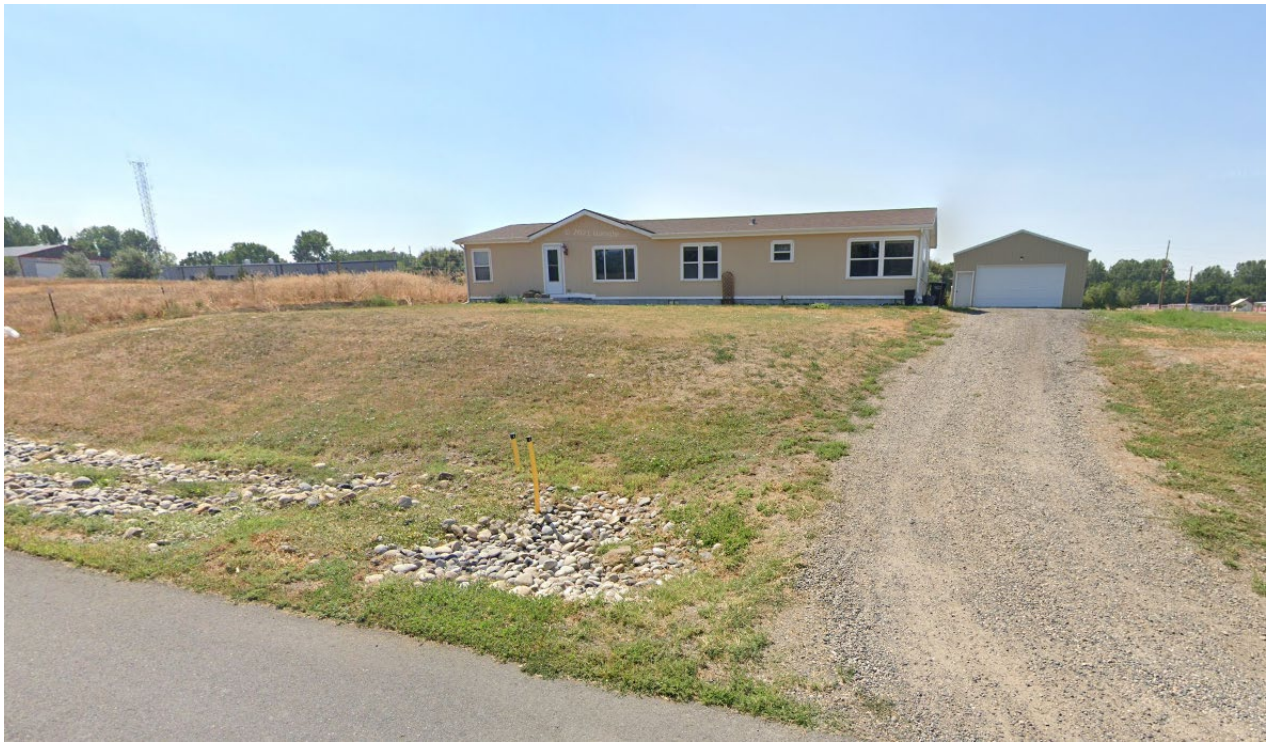
610 Mauser Street – dwelling on the south end of Lot 3
