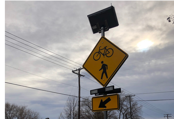
Rectangular Rapid Flashing Beacon (RRFB). Source: City of Billings
