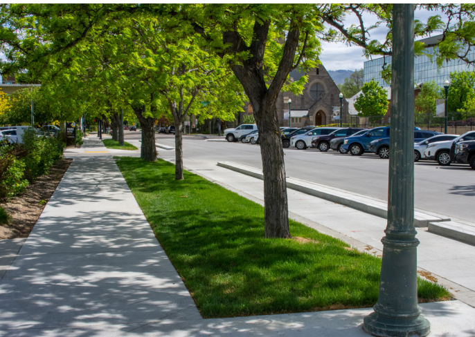
Separated bicycle lane. Source: Kittelson & Associates, Inc.
