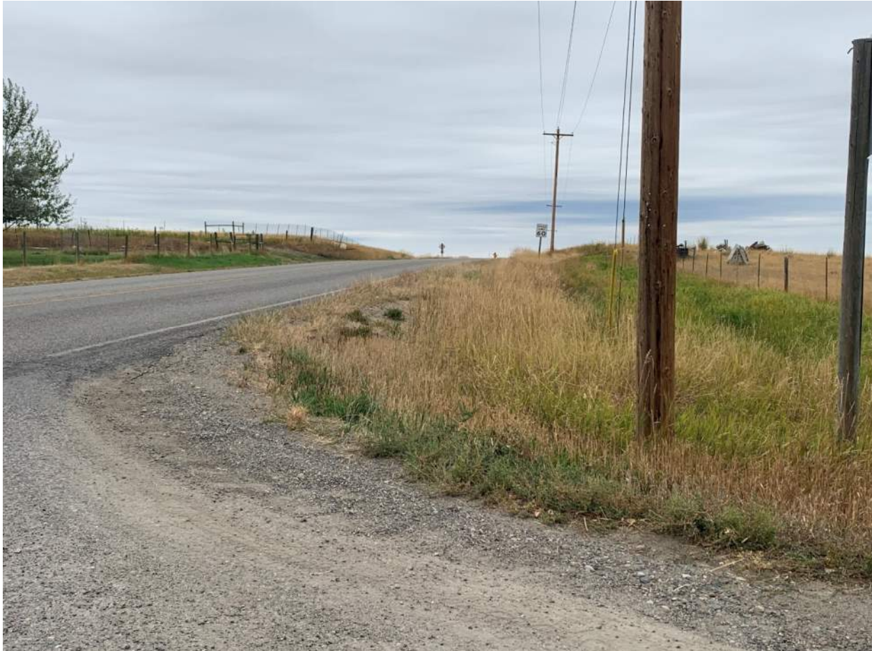
Figure 10: Field Measurements (Westbound, looking North at 610-feet)
