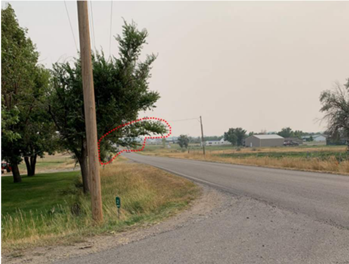
Figure 6: Tree Branch Obstructions (Westbound, looking South)
