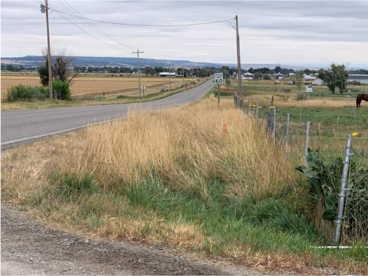
Figure 7: Field Measurements (Eastbound, looking South at 720-feet)
