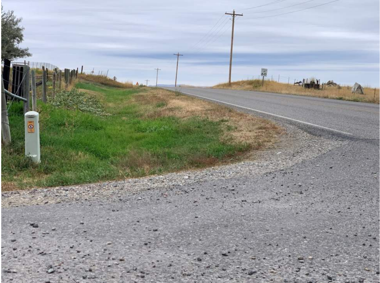
Figure 8: Field Measurements (Eastbound, looking North at 600-feet)
