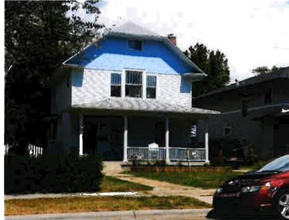
343 Clark Avenue (demolition)
