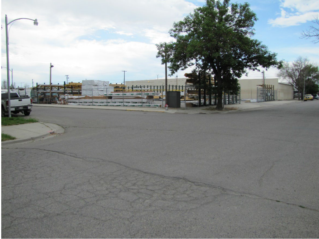
View to the southeast of subject property
