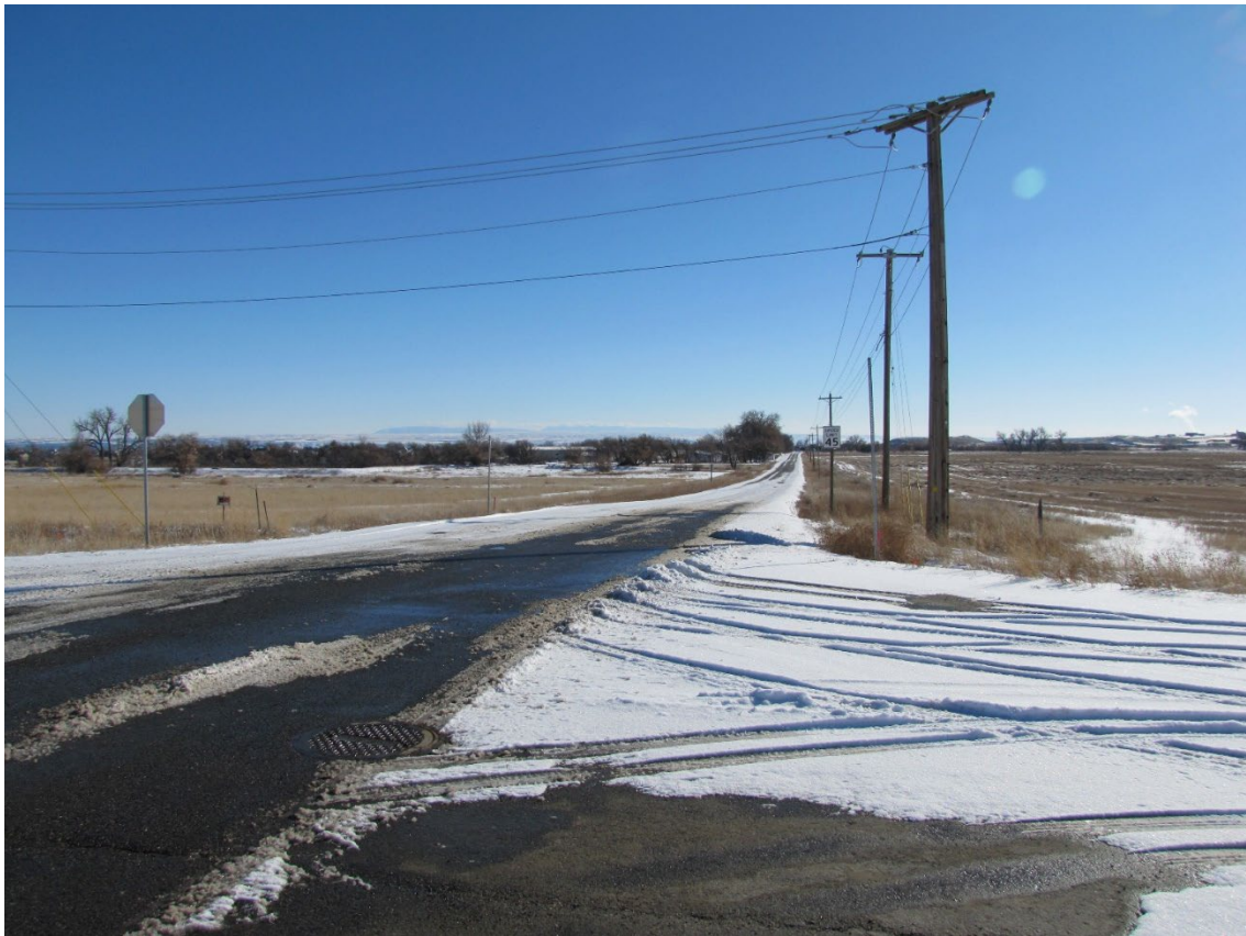
View south on 70 th St W
