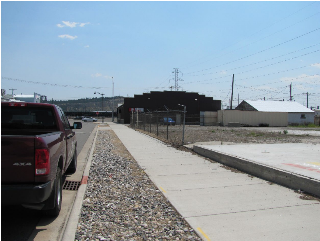
View south along N 12 th St
