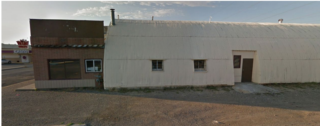
Billings Bronze Foundry on subject property prior to February 2018 fire
