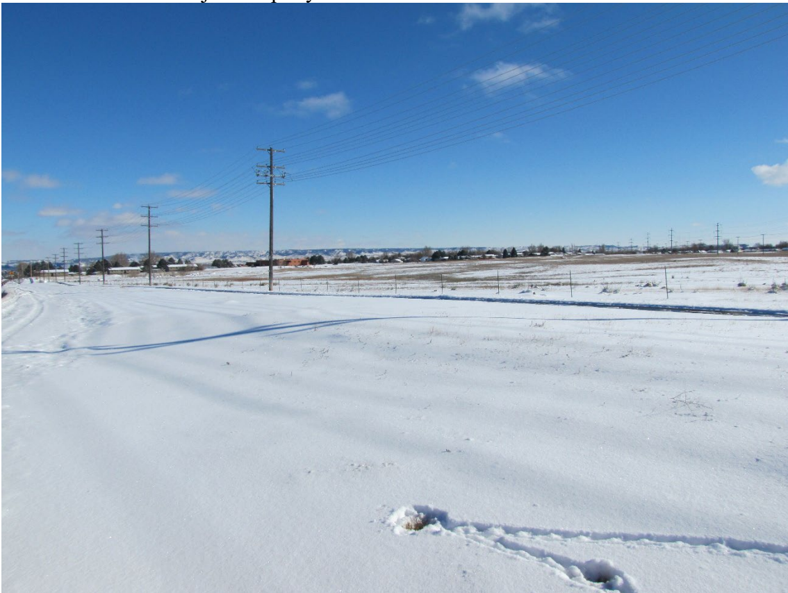
View south east along W Wicks Lane
