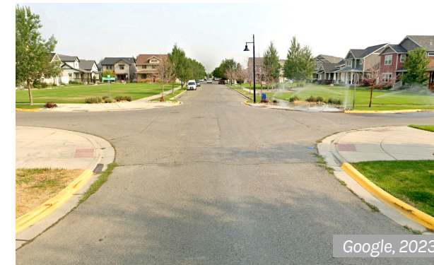
Curb extensions calm traffic in Josephine Crossing
