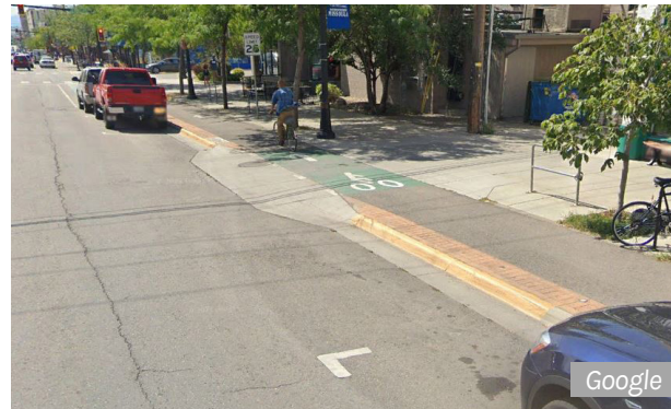
A protected bike lane at sidewalk level in Missoula, MT
