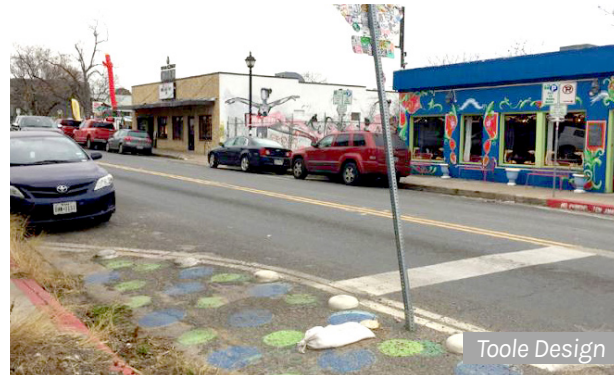
Easy-to-install materials such as paint, turtle bumps, and flex posts may be used to create curb extensions
