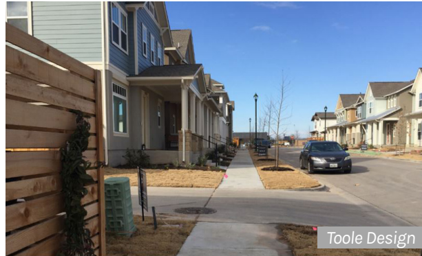
New sidewalk remains level across driveway
