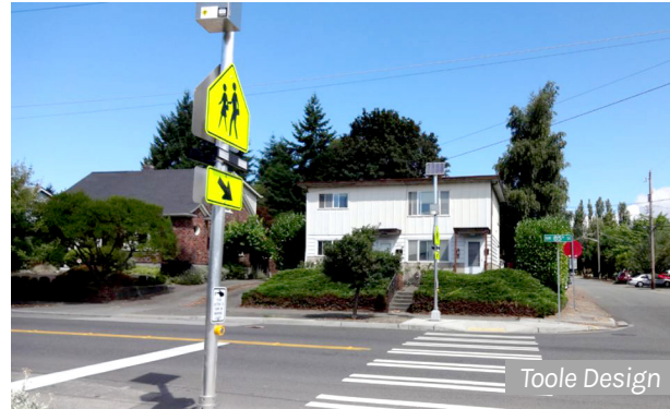
RRFB with push button at a school crosswalk
