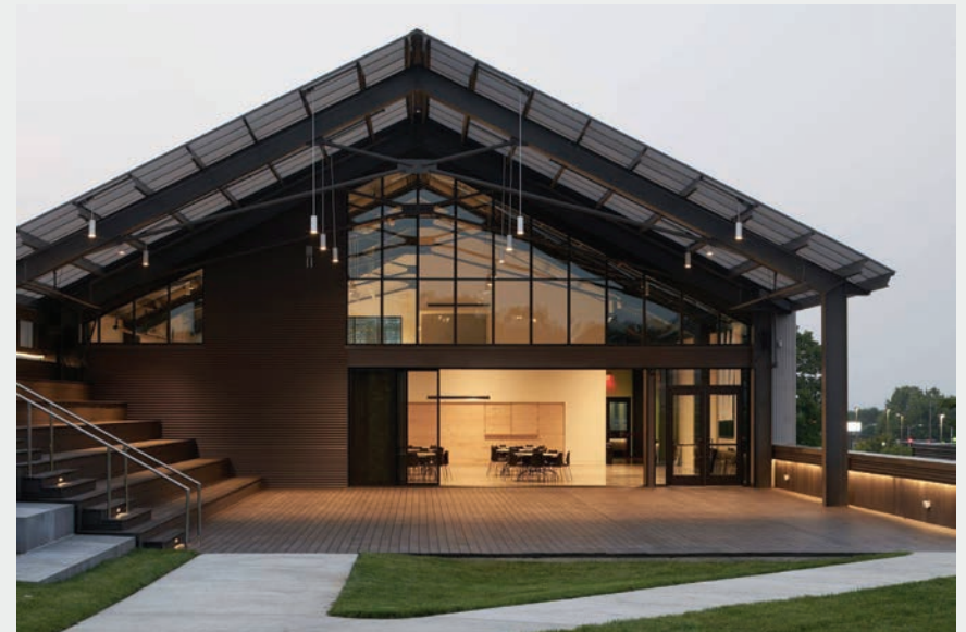
Figure 30. Example Community Center Building Metal Architecture. "HighlanderAccelerator_1.jpg.", https://www.metalarchitecture.com/articles/next-generation-community-center/
