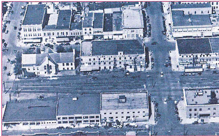
Above: An aerial view of Old Billings Hardware Building (center).
