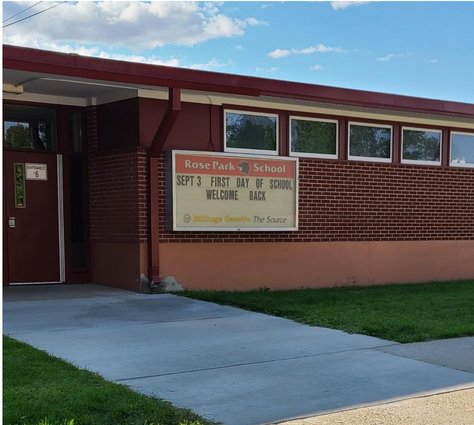
Existing message board
