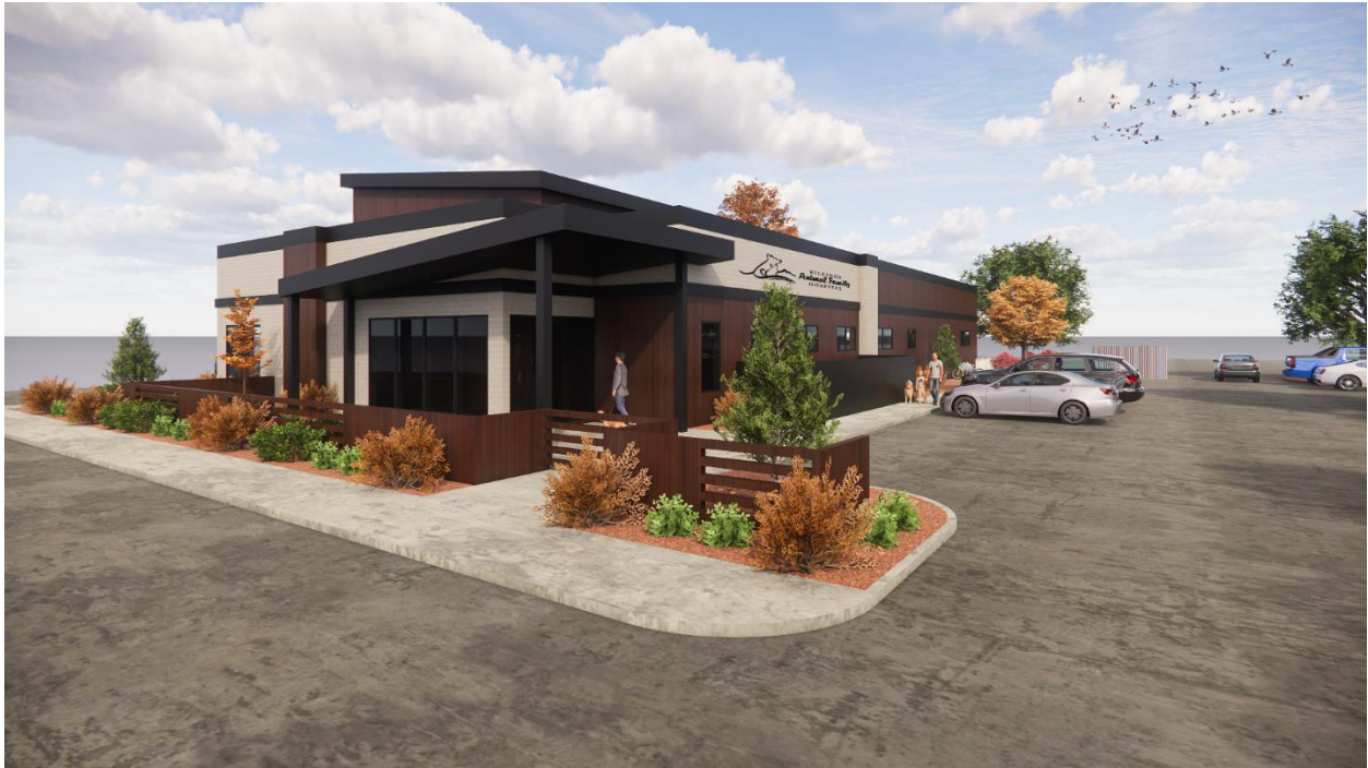
View from parking lot on East side
