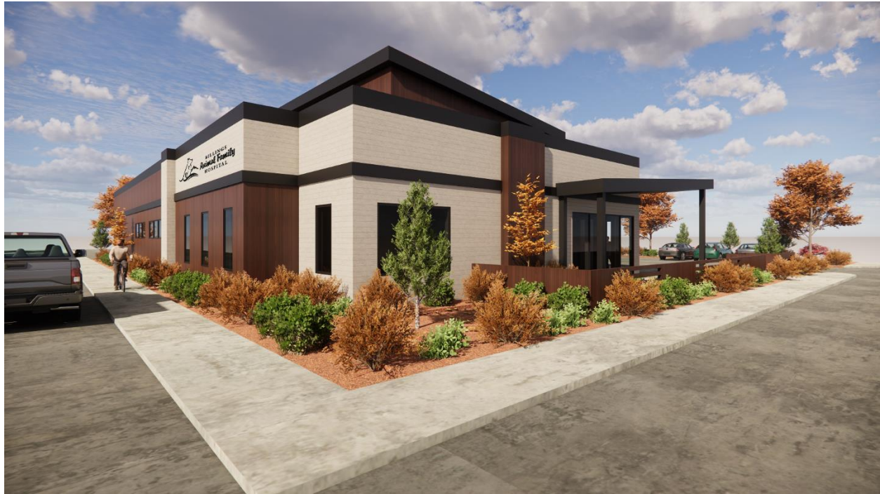
Street View from Corner
