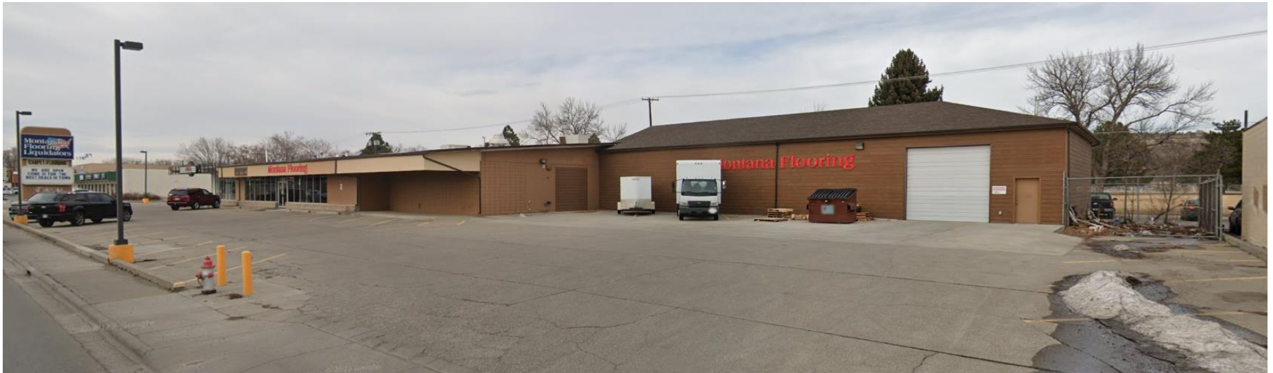
2135 Grand Avenue view northwest
