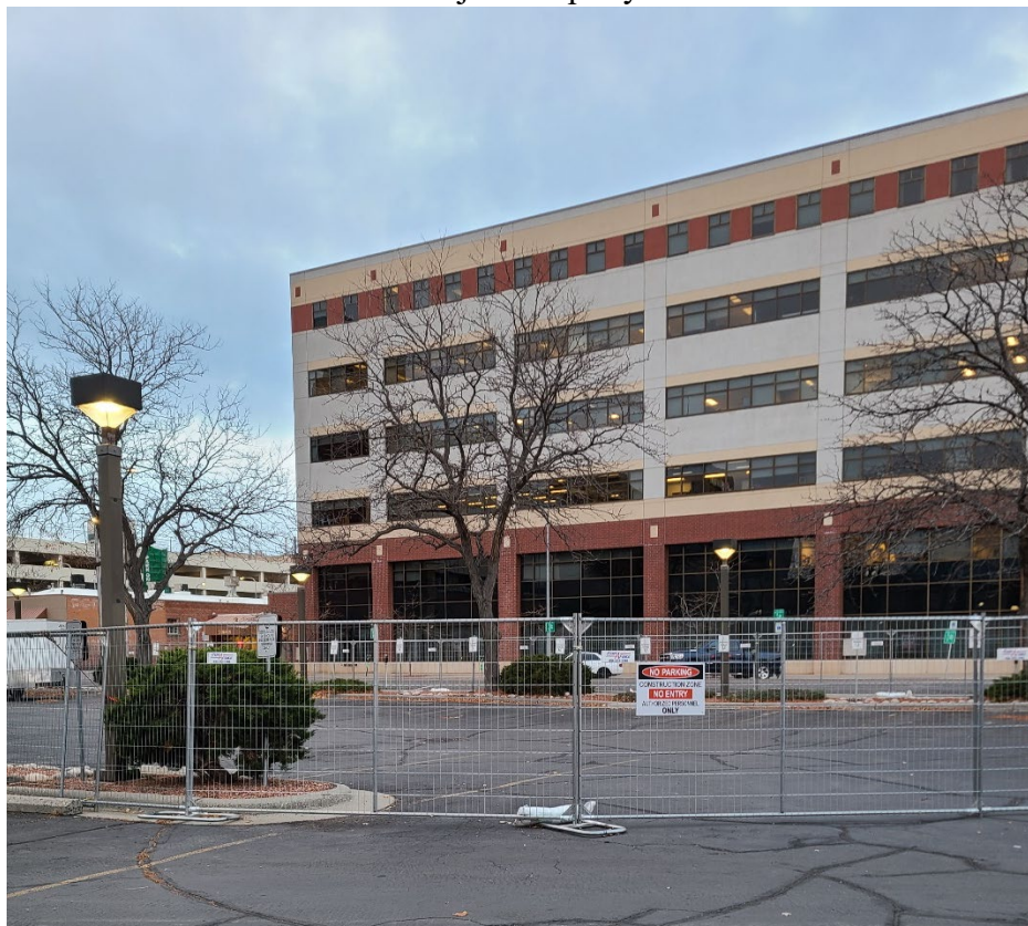
View south west across parking lot on 4 th Ave N
