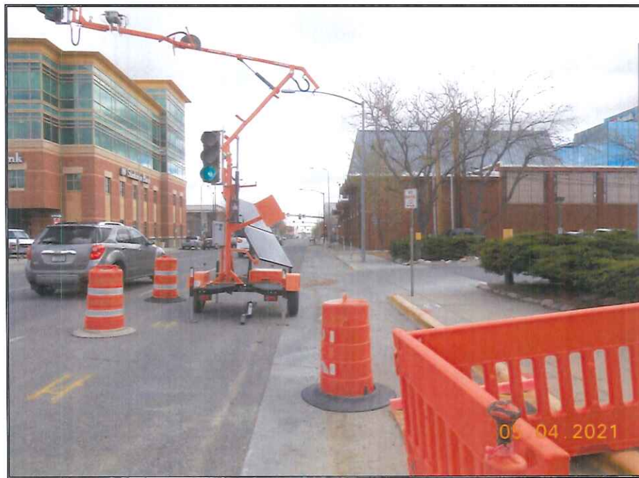
Looking to the northeast along the south side of 4 th Avenue North from near the northwest corner of the subject property. Taken by Matt Bender
