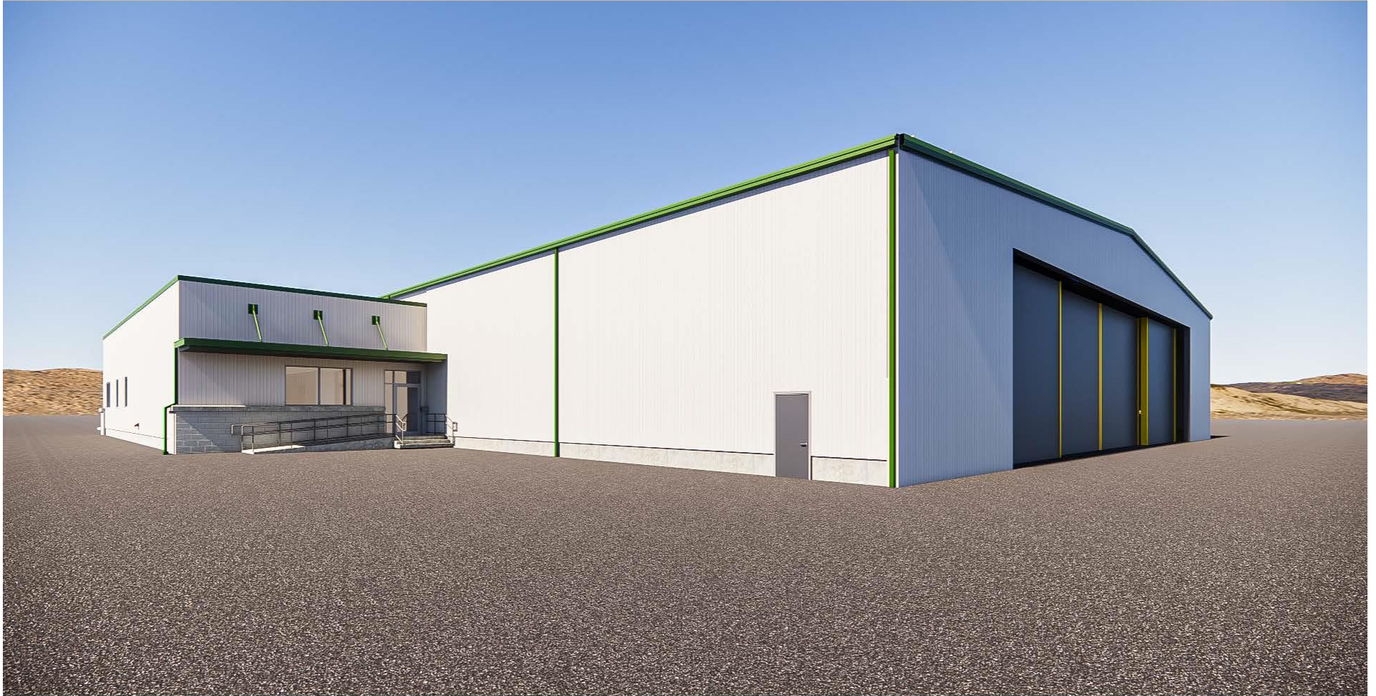
Aircraft Hangar & Office Bldg
