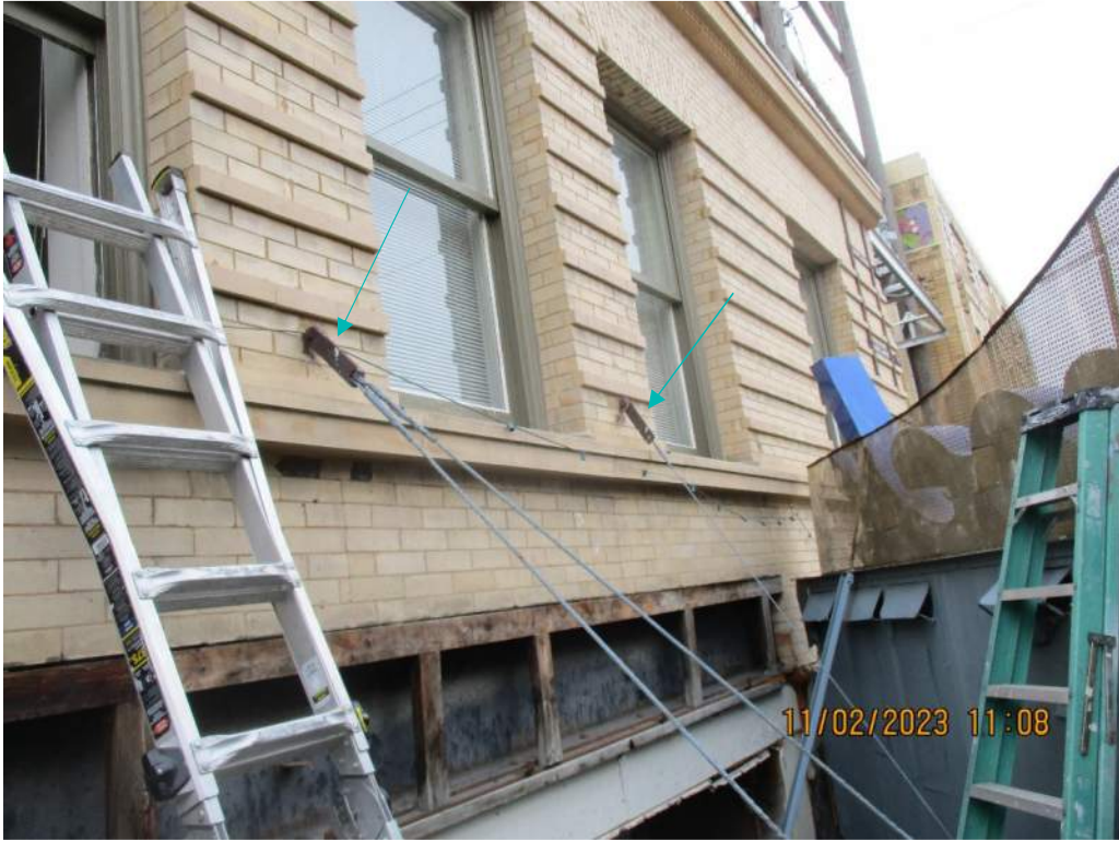
Figure 18: Cable Tie Back Connections at Exterior Wall
