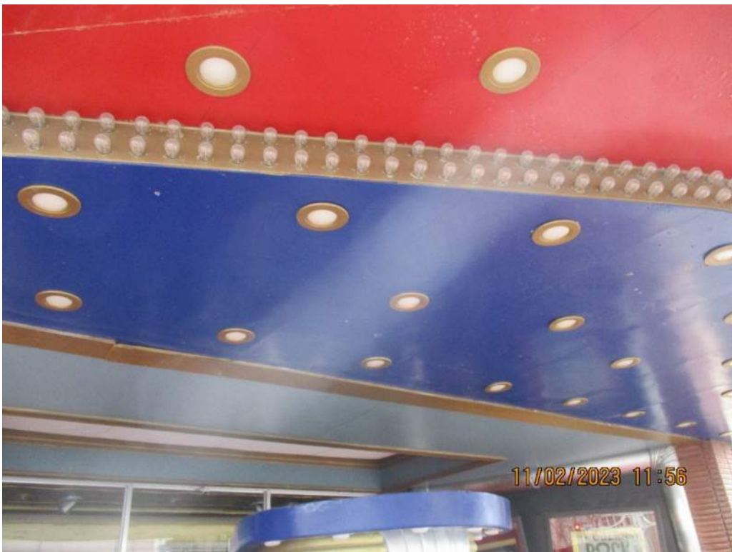
Figure 3: Overview of Babcock Theatre Marquee Underside
