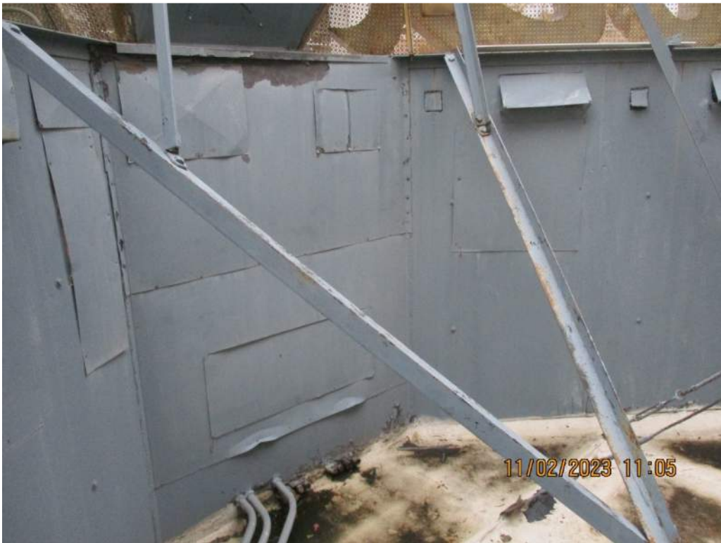
Figure 7: Overview of Marquee Interior North Side Metal Paneling
