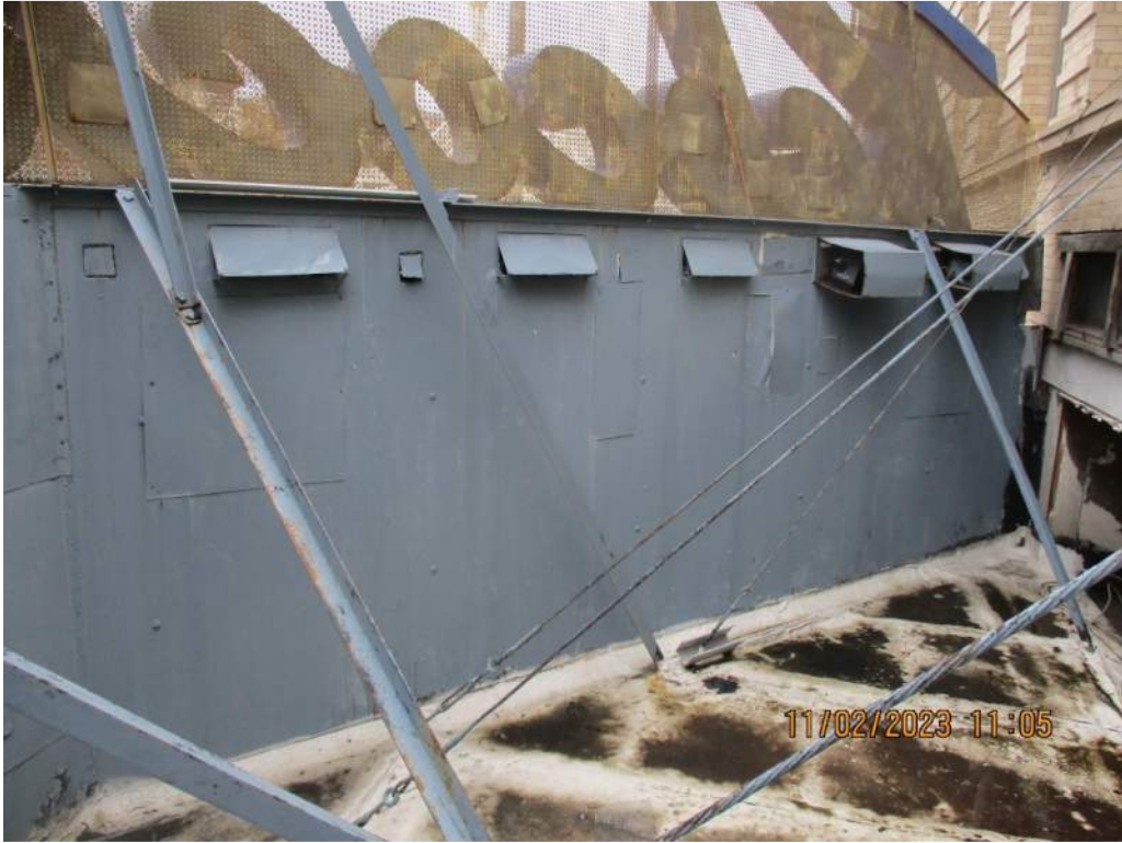
Figure 6: Overview of Marquee Interior East Side Metal Paneling
