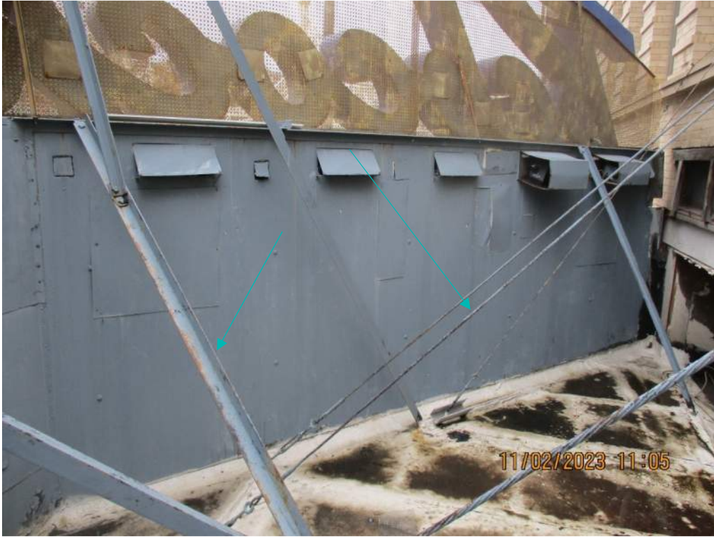
Figure 16: Marquee Support Cabling and Angle Iron Bracing
