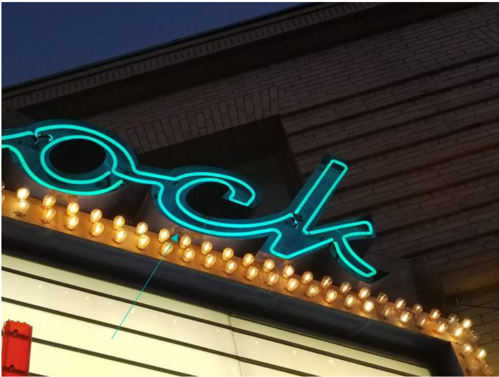
Figure 23: Observed Deterioration at Underside of "Babcock" Lettering
