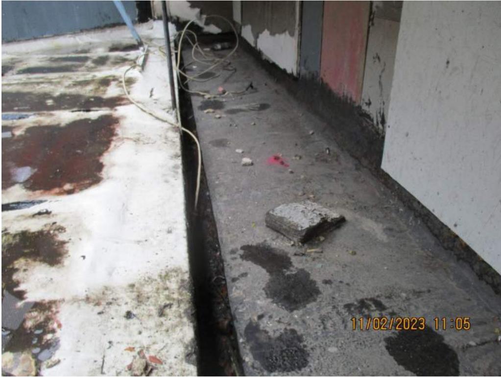
Figure 12: Internal Gutter Underneath South Wall of Marquee
