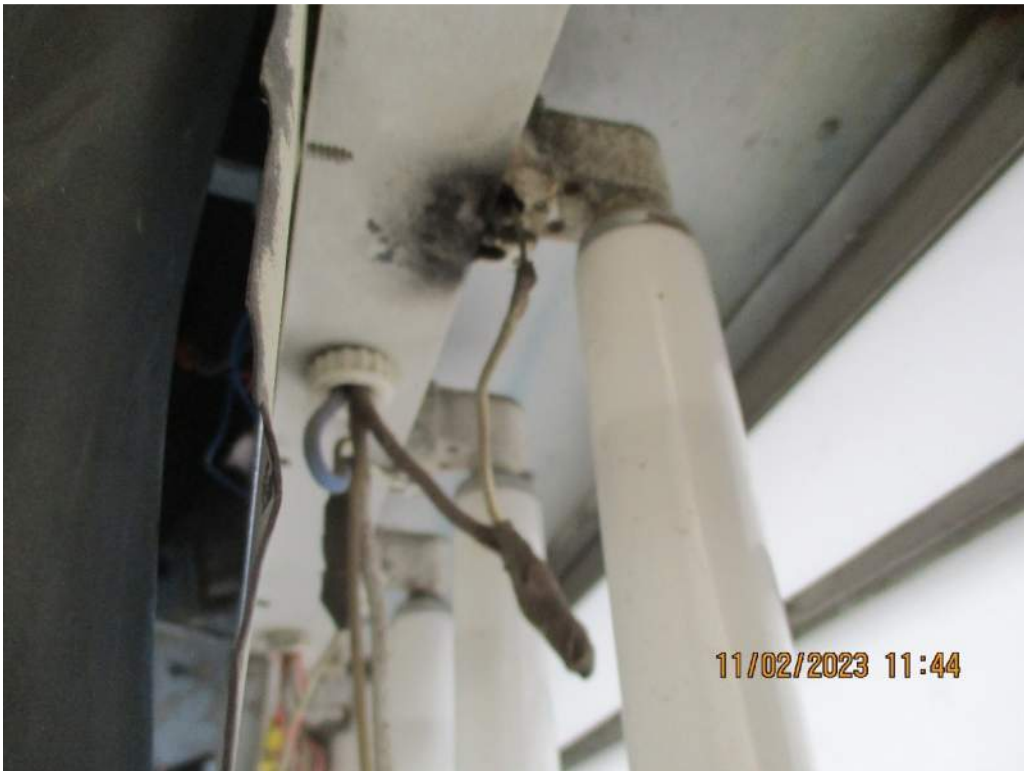
Figure 21: Interior Lighting Withing Exterior Paneling of Marquee
