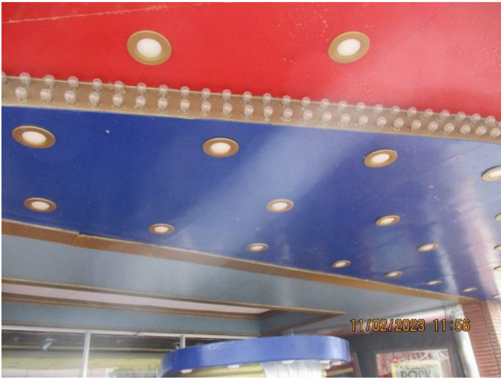
Figure 3: Overview of Babcock Theatre Marquee Underside
