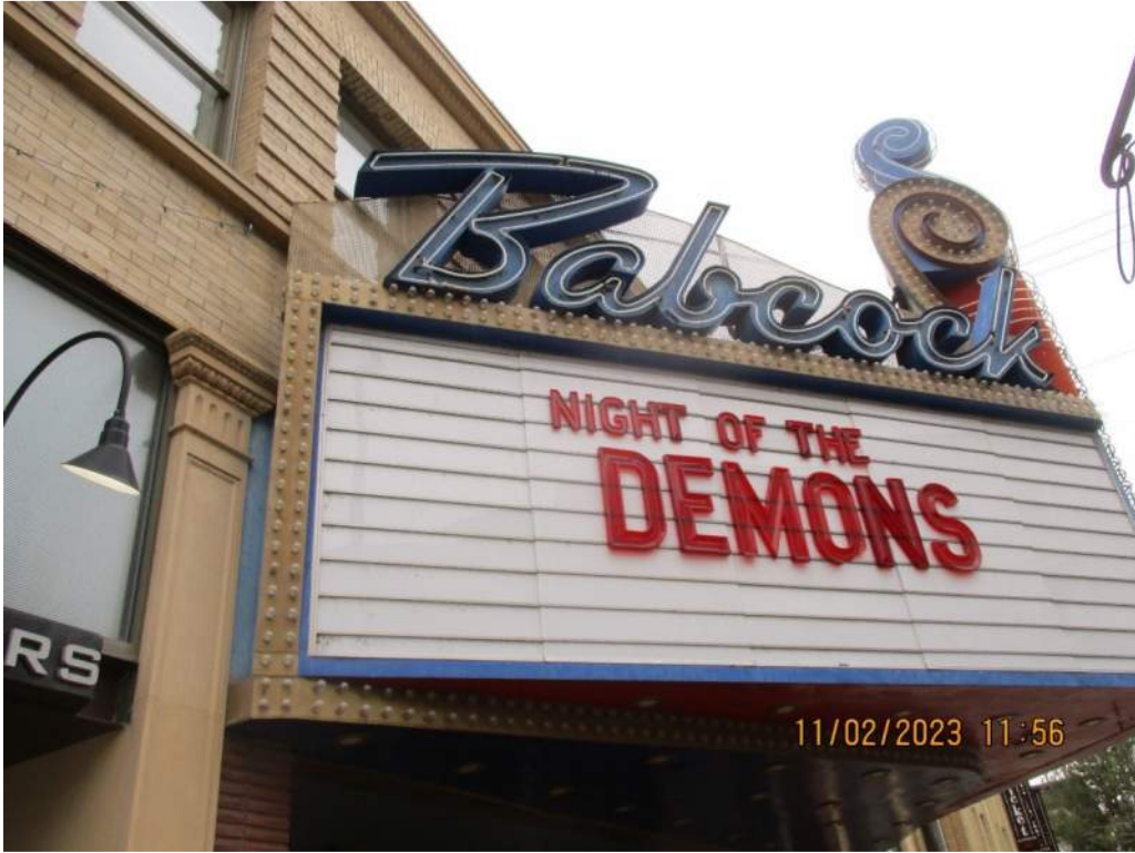
Figure 2: Overview of Babcock Theatre Marquee from Street
