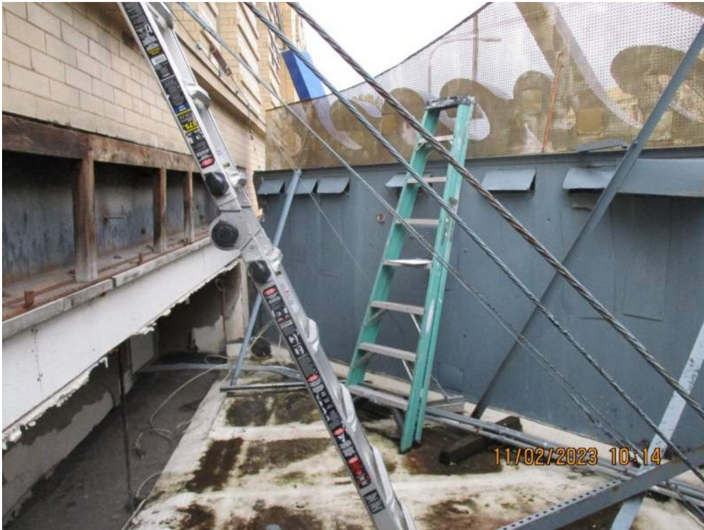
Figure 8: Overview of Marquee Interior West Side Metal Paneling
