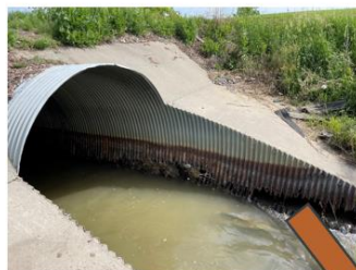
Corroded Culverts
