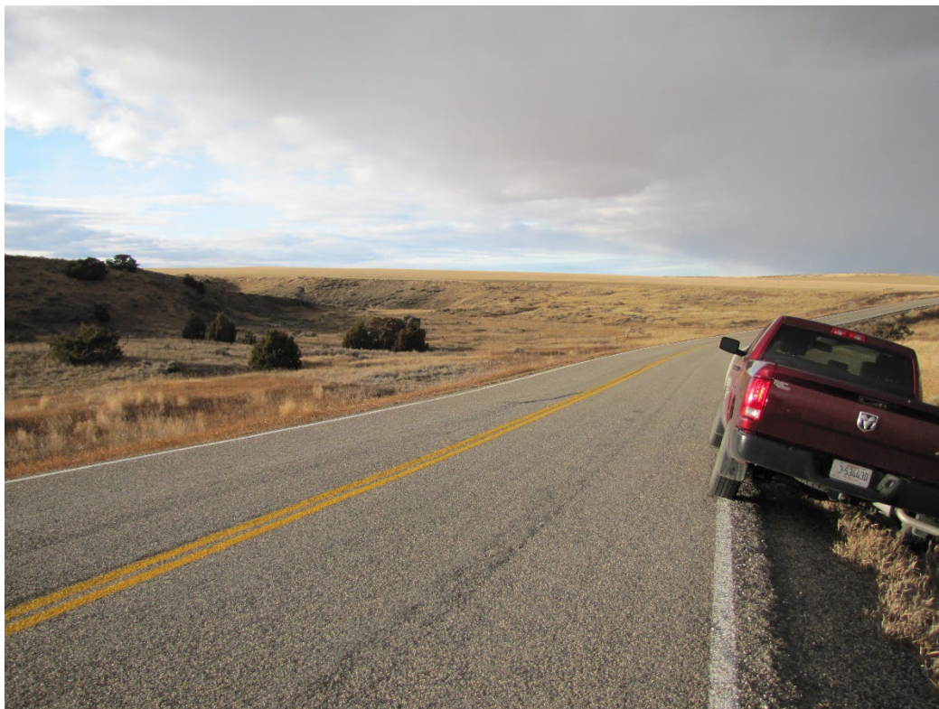
View north on Collier Rd
