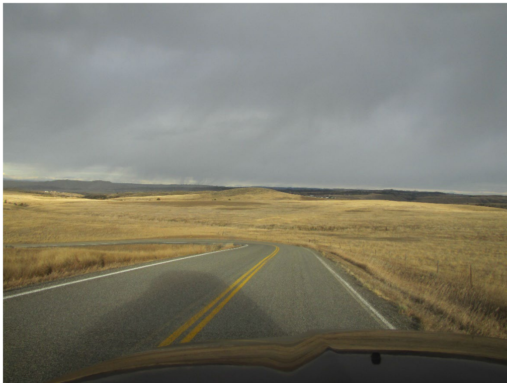
View north and east on Collier Rd
