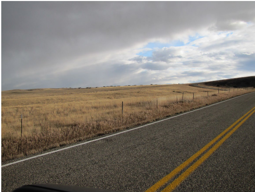
View south and east from Collier Rd
