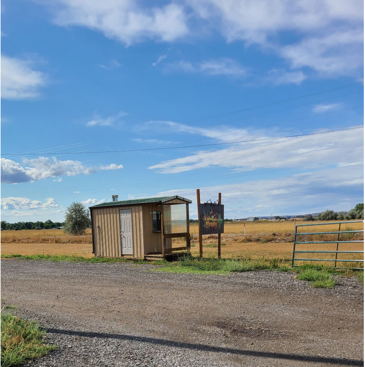
Secondary structure on subject parcel
