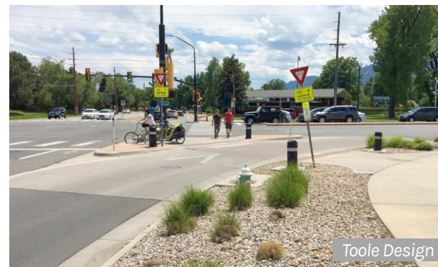
Slip lanes with added signs and raised crosswalks bring attention to pedestrians
