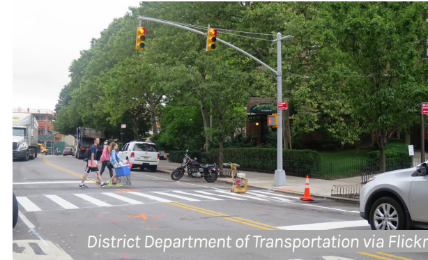
Mid-block crossing with traffic signal
