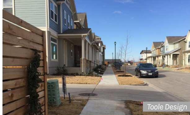
New sidewalk remains level across driveway
