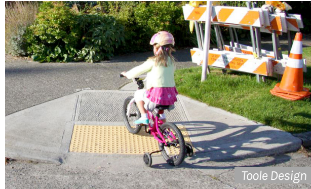
A sidewalk retrofitted with a curb ramp and a tactile warning strip
