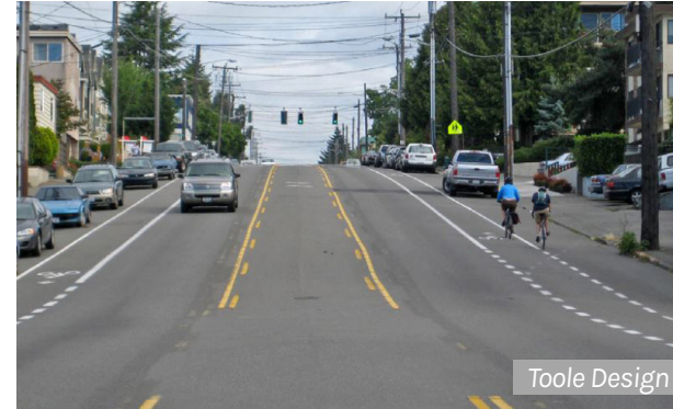
Center turn lane narrowed to provide space for bike lanes
